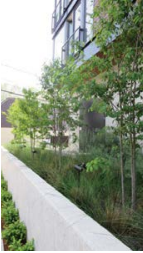
at grade bioretention planter
