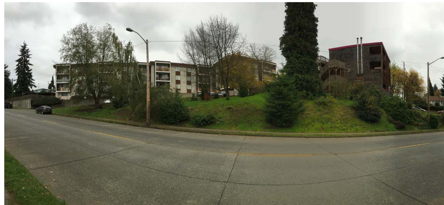
SITE FROM WEST
