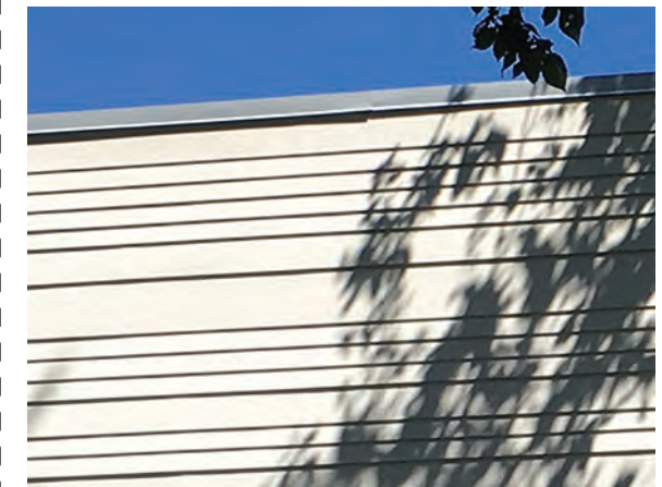
Varied widths of lapped fiber cement siding
