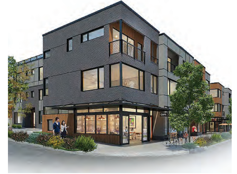
RALLY LIVE-WORK UNITS - JOHNSTON ARCHITECTS - Large operable windows facing California Ave SW - Stepped facade defines individual units and creates visual interest at street-level - Glass canopy provides overhead weather protection at the corner
