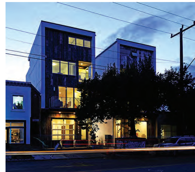
3237 CALIFORNIA AVE SW - DWELL DEVELOPMENT - Glazed garage door at the street-level - Progression of entry elements; patio provides buffer at street edge and doors protected by deck overhang above
