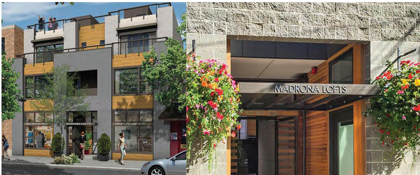
MADRONA LOFTS - DAVID VANDERVORT ARCHITECTS - Use of different CMU finishes to detail the entryway - The signage is integrated with the fenestration - Layer of secondary elements to provide a human scale to the street-edge such as hanging planters
