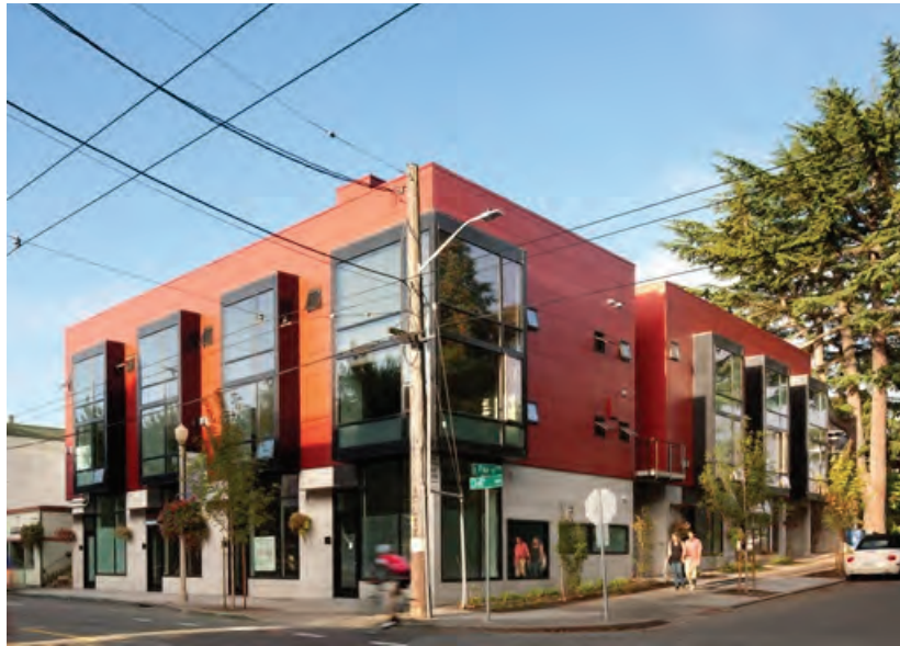
PIKE STATION - ATLIER JONES - Corner accentuated by bay window - Division of materials highlights live-work uses - Units divided between two separate buildings; reads as a single mass with identical details at each elevation
