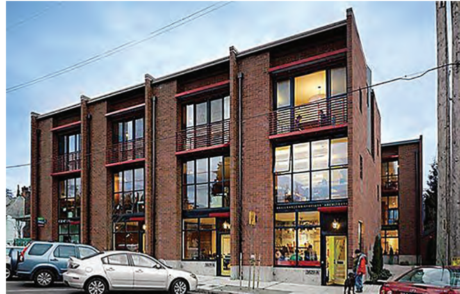
COLUMBIA CITY LIVE-WORK UNITS - PHILIP CRISTOFIDES - Appropriate use of masonry - Shallow balconies along street edge - Different treatment of fenestration at each floor level
