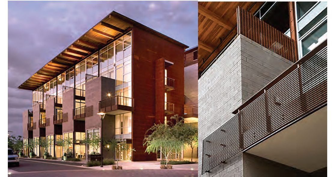
SAFARI DRIVE CONDOMINIUMS - MILLER HULL - Combination of CMU block and weathered steel - Deep decks above the entries are recessed between opaque massings to create privacy
