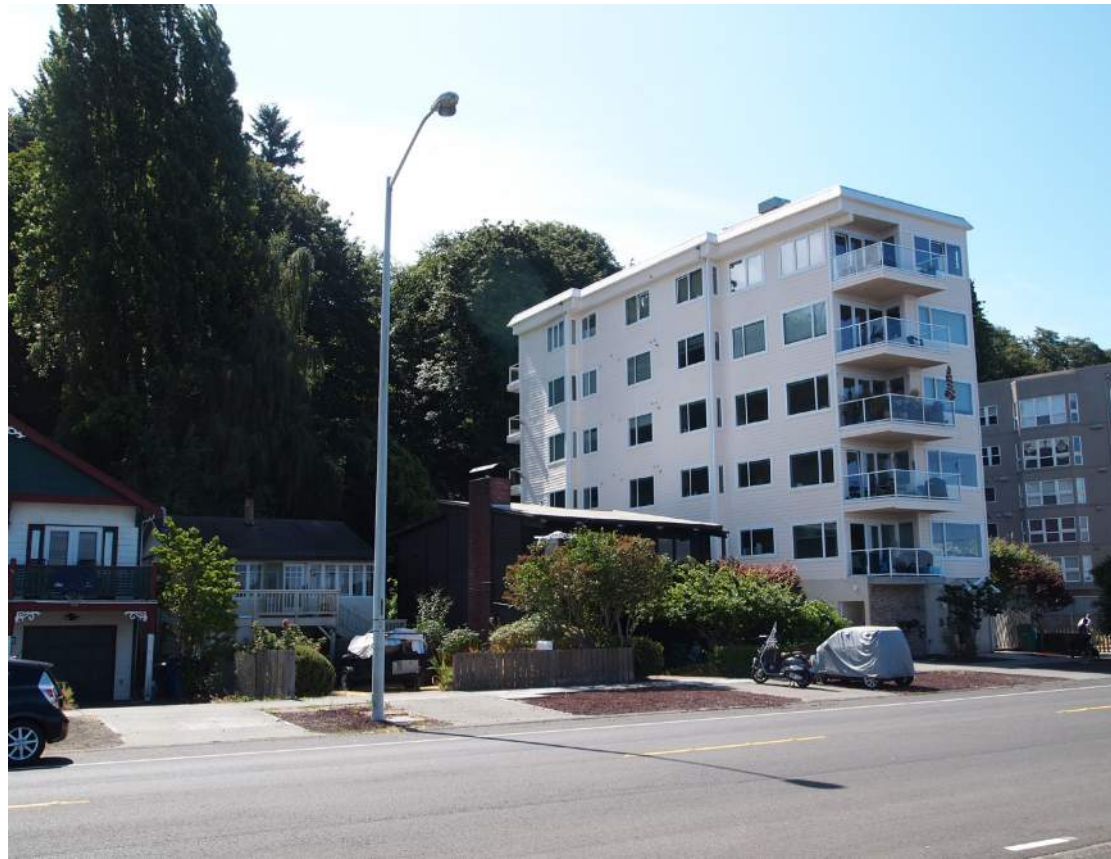
VIEW OF PROJECT SITE WEST EDGE
