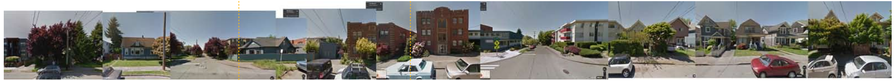
12th Avenue E - West Elevation Smaller existing structures to the north, 3 story brick apts & single family house across from site
