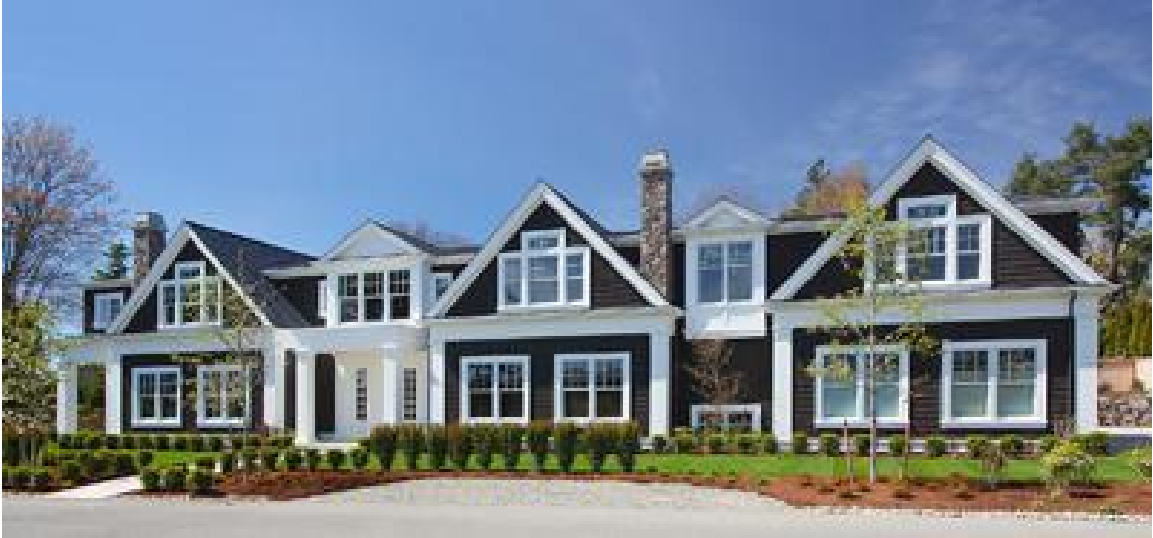
Medina Private Residence (Landmark Property Holdings)
