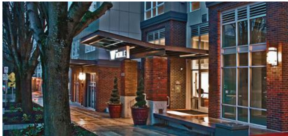
Adequate lighting and visibility to the outside (PL2.B)
