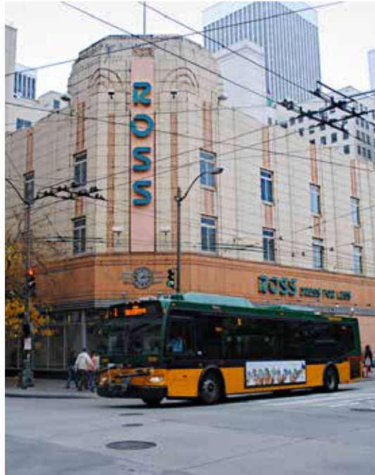
1940 / 45' / 3 Floors / Office & Retail
