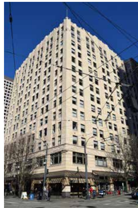
1929 / 160' / 14 floors / Office & Retail
