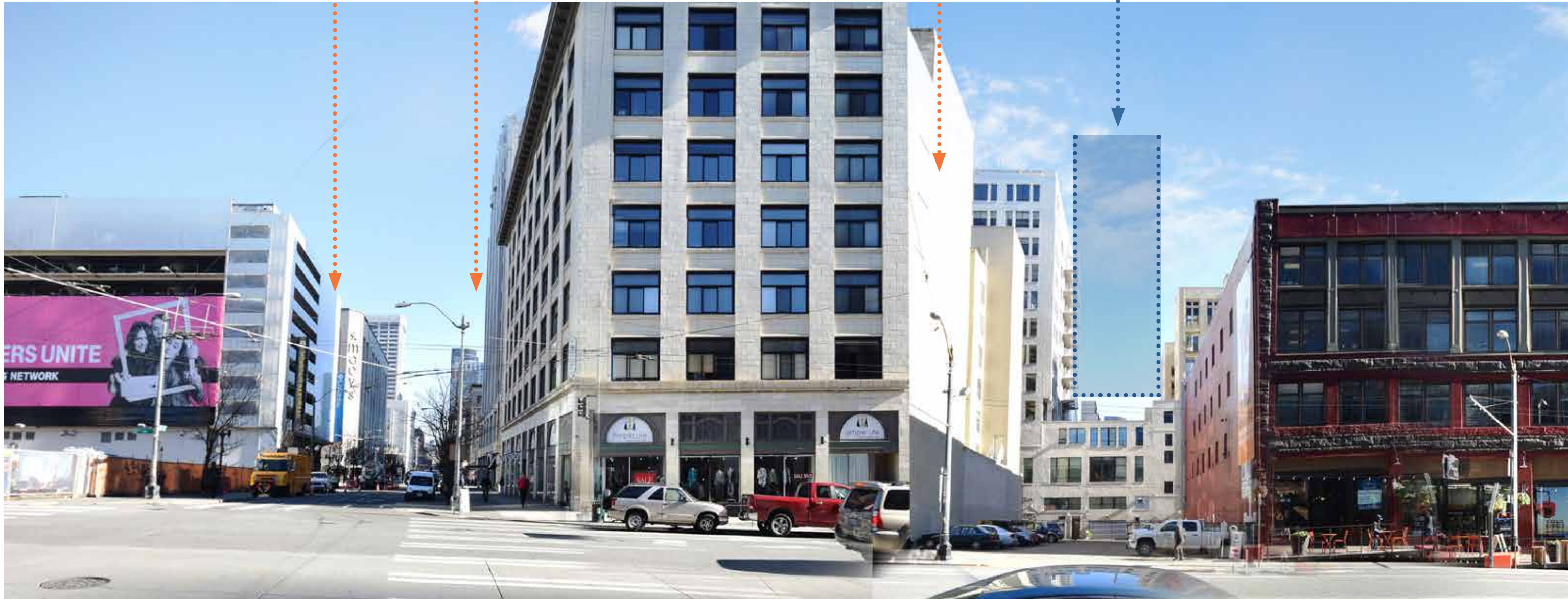
16 2nd + Pine Future Tower Site 3rd Ave. Garage/Columbia Sportswear Beyond
