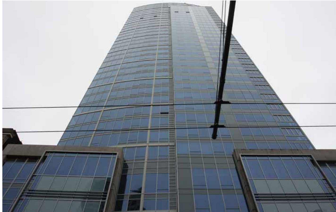
The 440' tall, taut glass skin tower looms over the block. Transparency is not apparent from street perspective as glazing is reflective and blue tint is pronounced.
