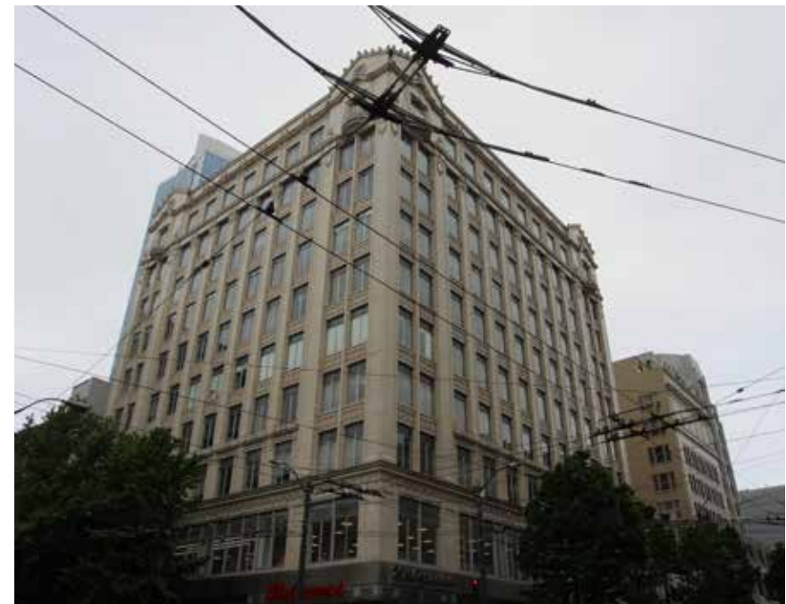
1928 / 125' / 11 floors / Office & Retail
