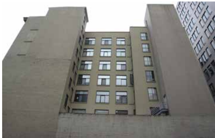
Existing void at Haight Building (north site edge)
