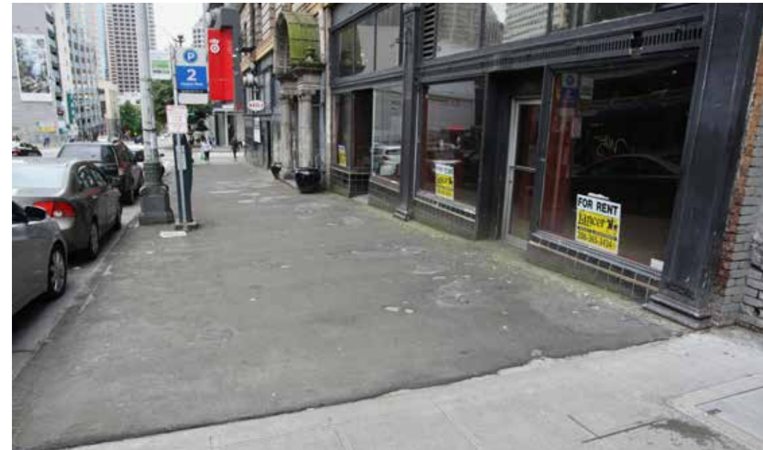
Sidewalk is mix of materials and textures including concrete, asphalt, moss and pigeon droppings.
