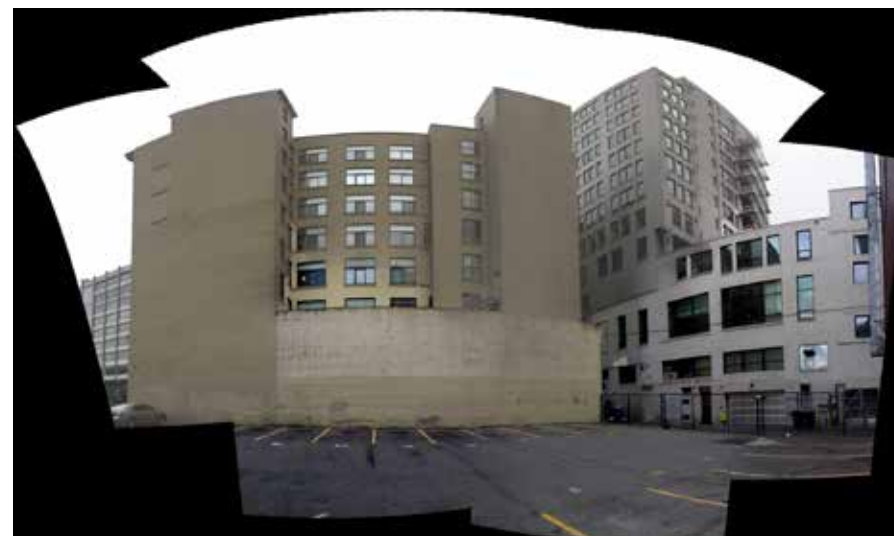
Haight building south facade
