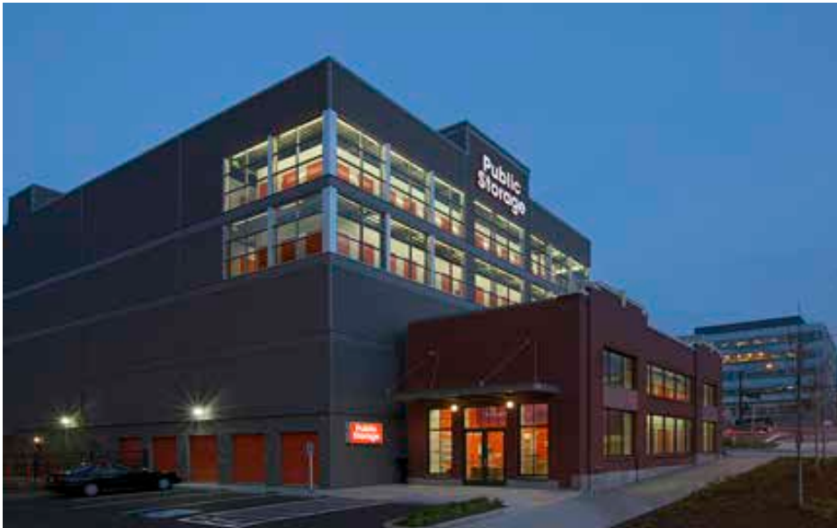
Nighttime lighting emphasizing storage building's internal function
