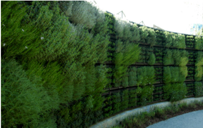
Greenwall in grid pattern using modular system
