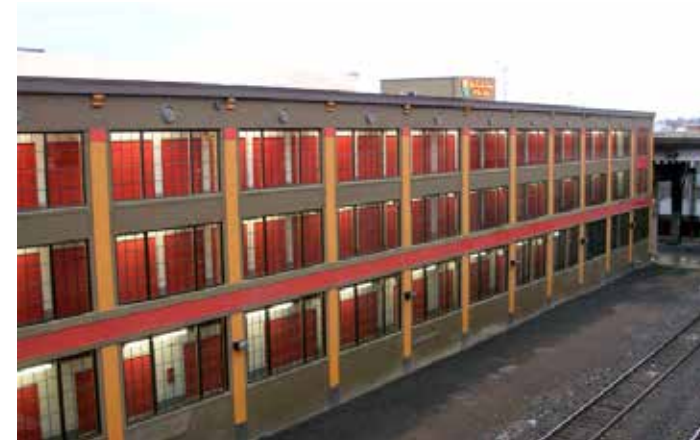
Storage corridors visible through storefront
