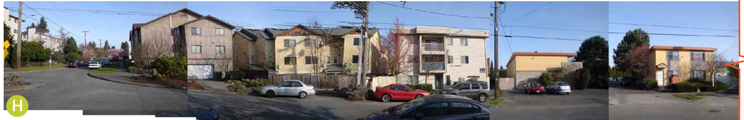
View of residential structures across N 95th Street looking North.
