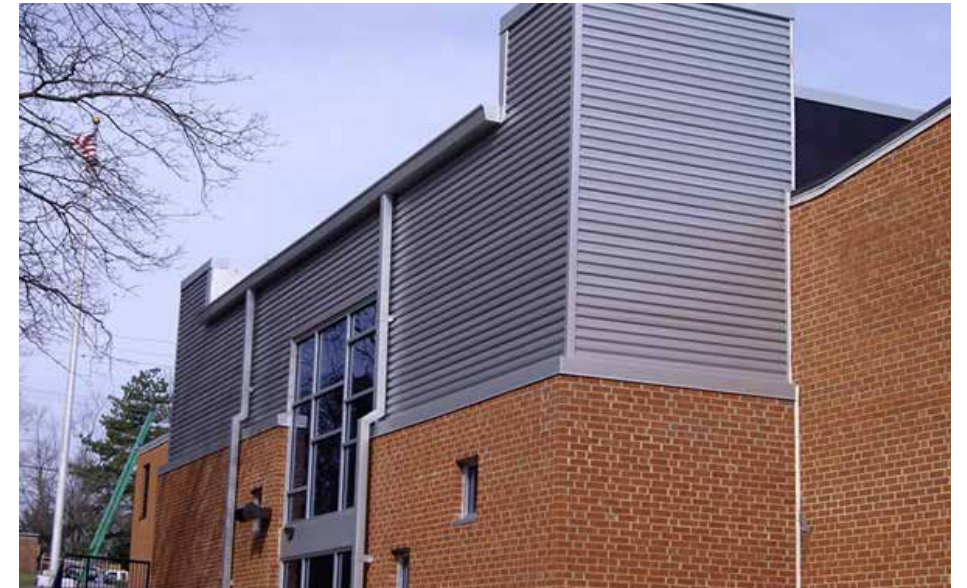
Finish material contrast with brick and metal siding
