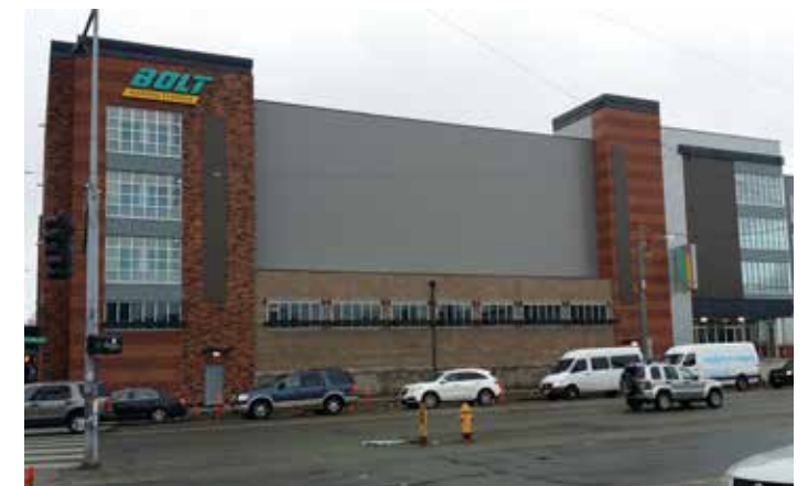
Contemporary self-storage building using materials and modulation to reduce apparent bulk
