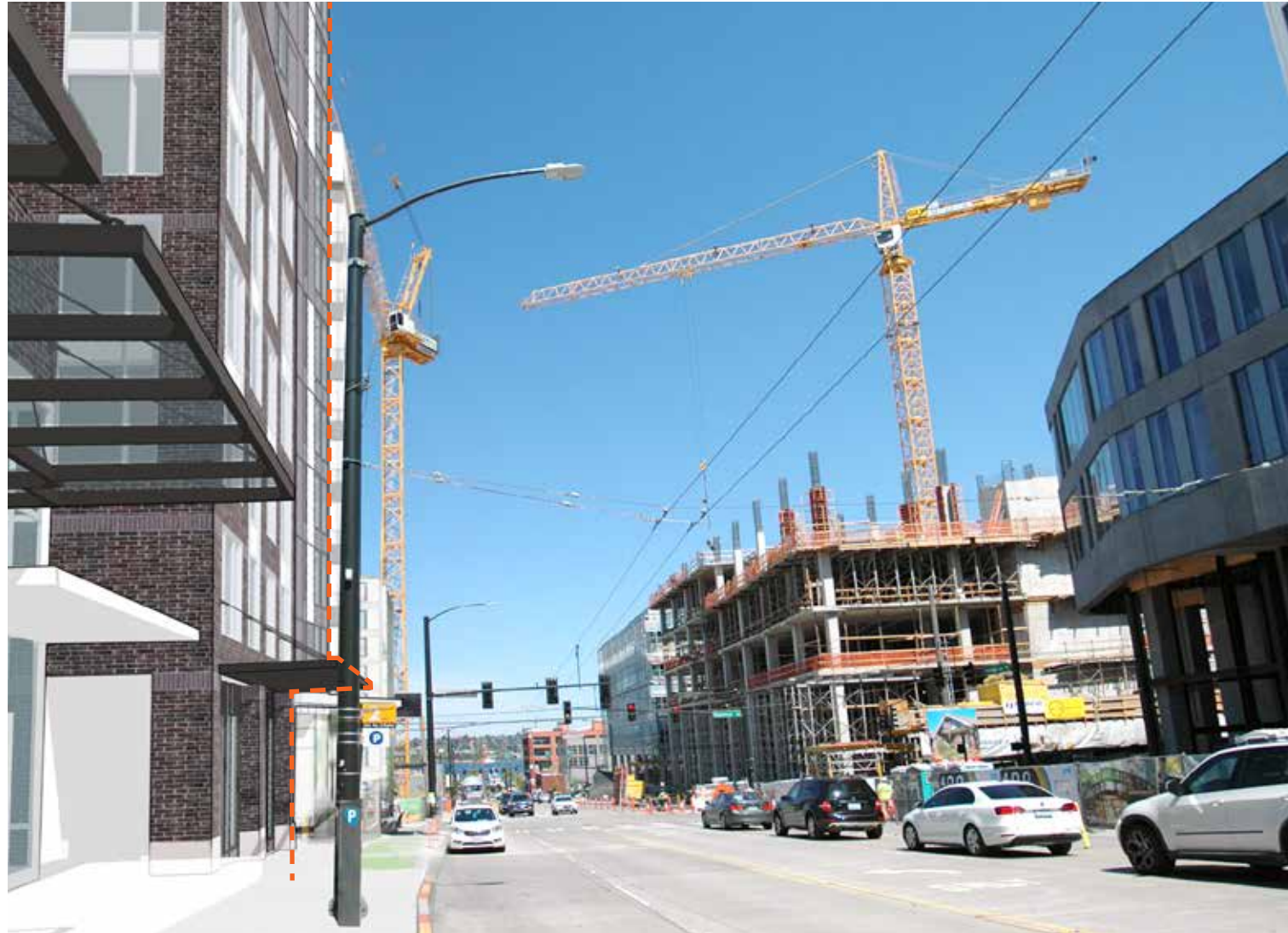
1 VIEW AT PROJECT SITE ON FAIRVIEW AVE N
