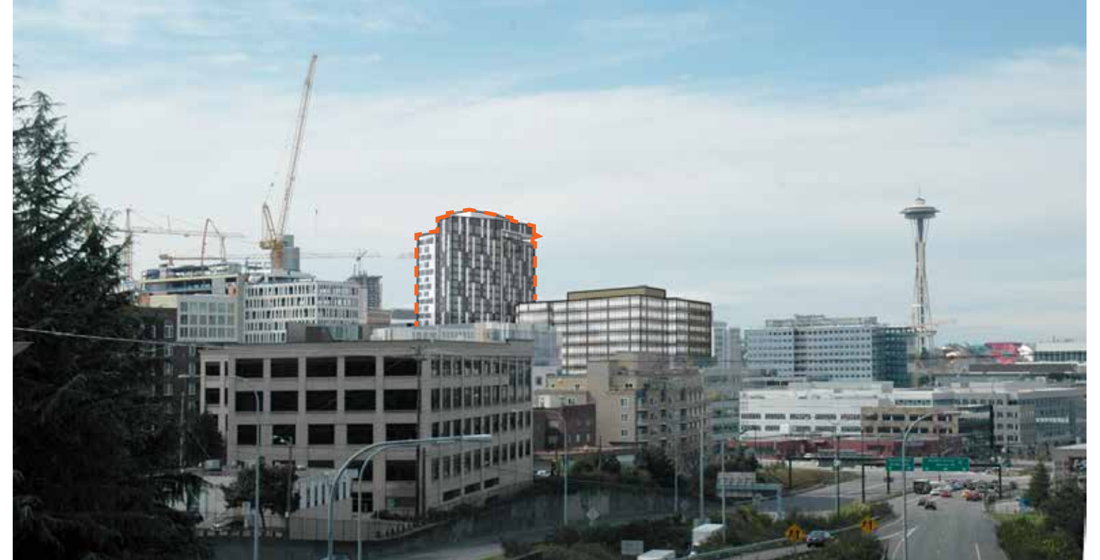
VIEW FROM EASTLAKE AVE E TO THE NORTHEAST OF PROJECT SITE
