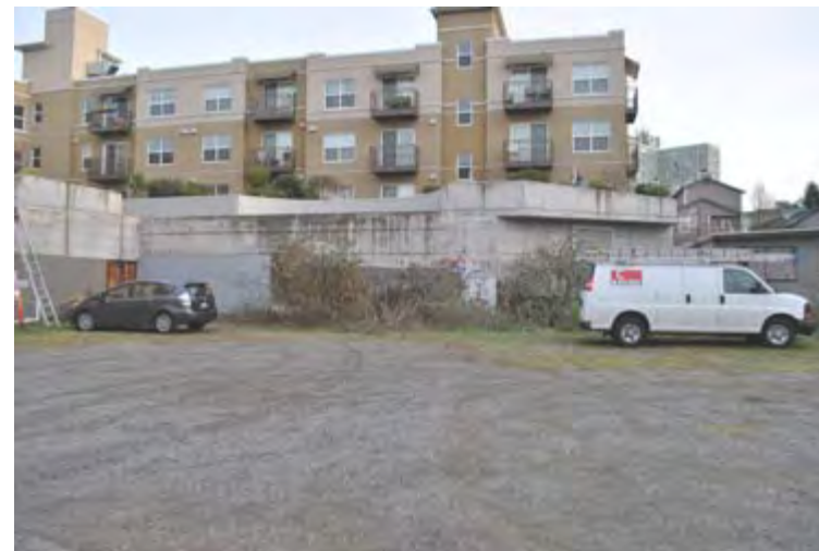
4 Florera Retaining Wall - Looking East
