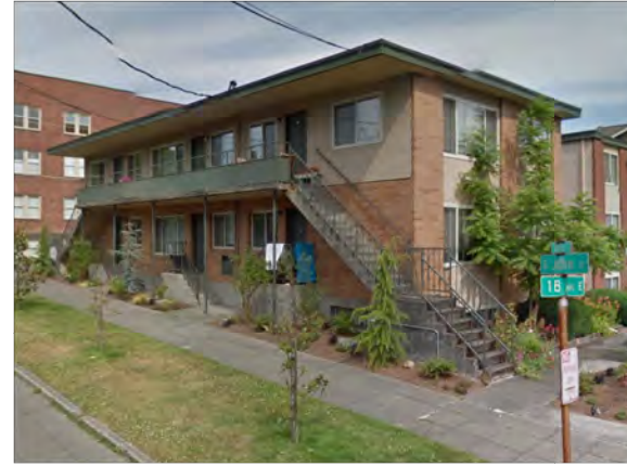
⑧ APARTMENT BLDG. - 1720 E. JOHN ST.
