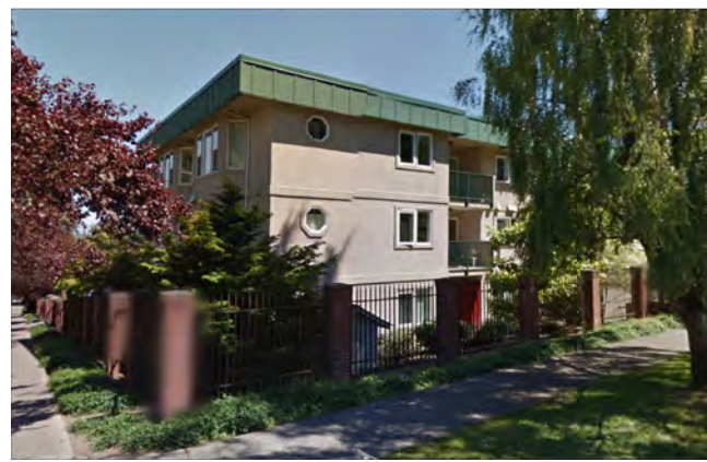
② APARTMENT BLDG. - 1819 E. DENNY WAY
