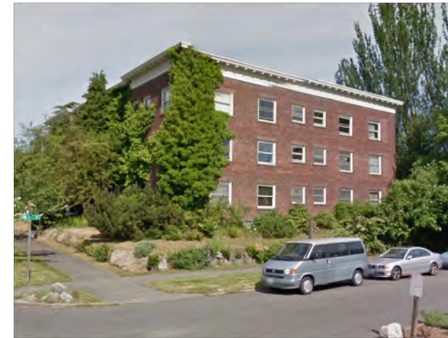
⑥ APARTMENT BLDG. - 1720 E. DENNY WAY
