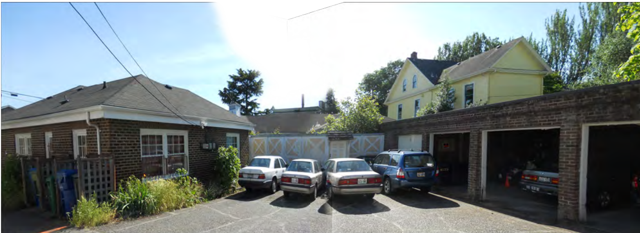
⑤ EXISTING PARKING FROM ALLEY LOOKING EAST
