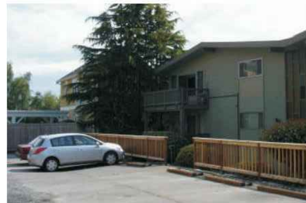
I:View Alley looking South West(Johnston Manor alley parking)
