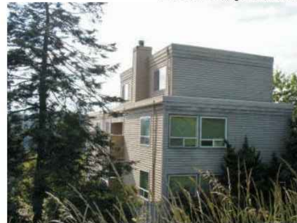
E: View 14th ave looking west
