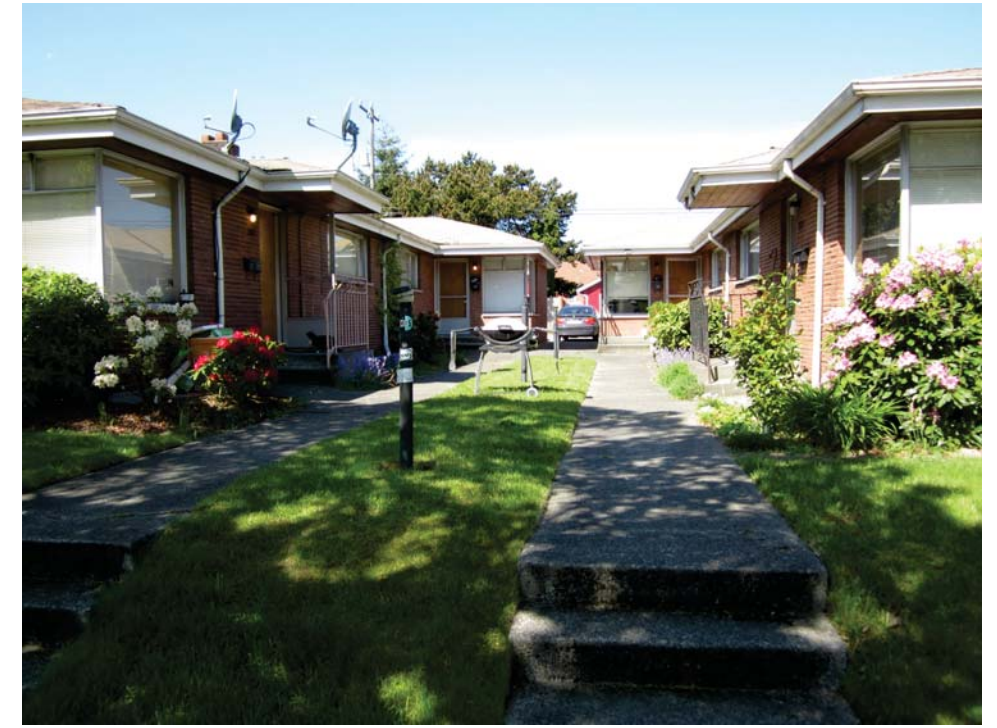
2. LOOKING WEST FROM CALIFORNIA AVE SW
