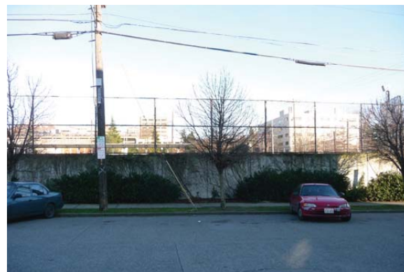
12. Seattle University Playing Fields with Eight Foot Retaining Wall
