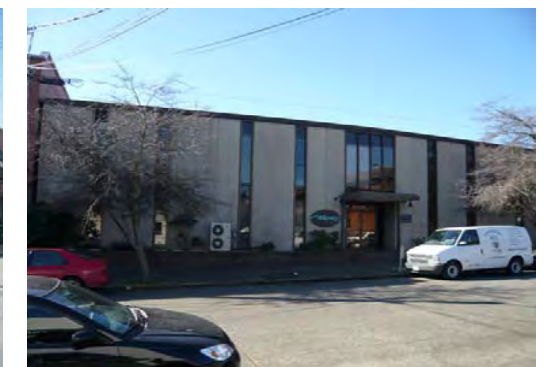
14. 2 Story Office Building
