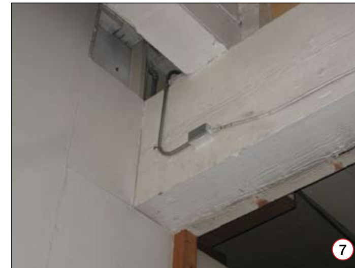
BEAMS IN EXISTING BUILDING TO BE SAVED
