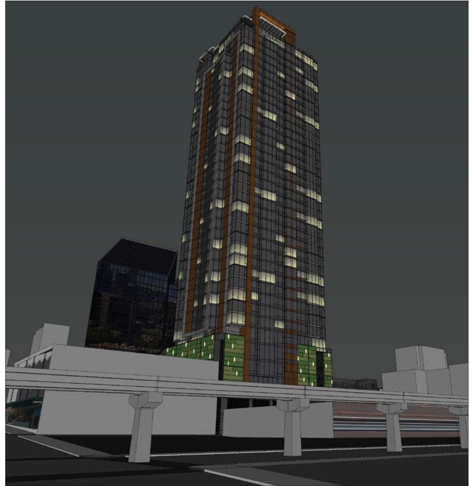
TOWER VIEW LOOKING FROM SOUTHEAST
