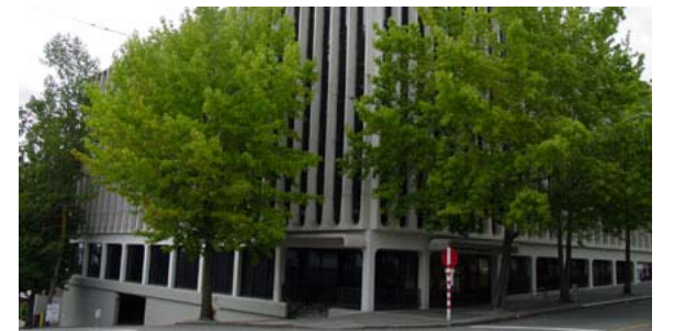
W HARRISON ST PLAZA BUILDING
