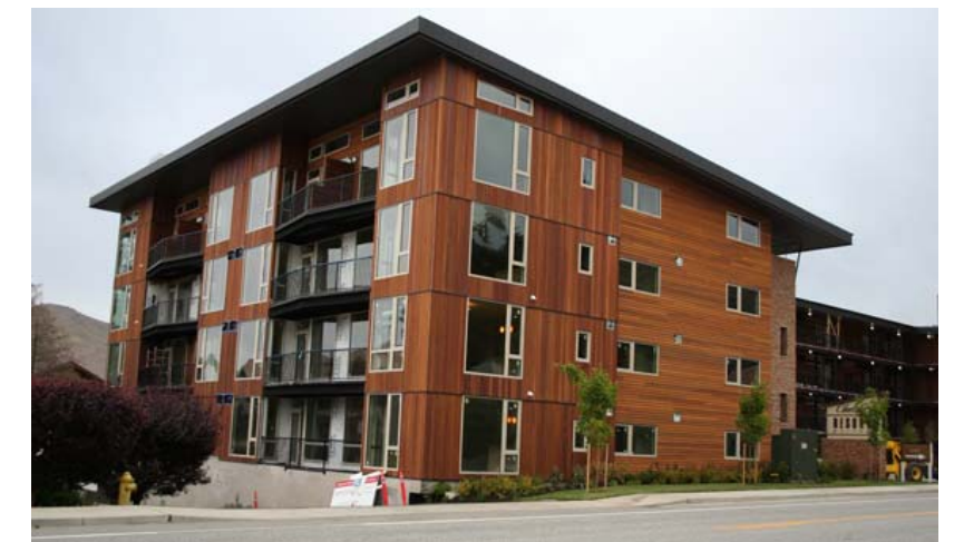
Chelan Resort Suites Completed Spring 2007
