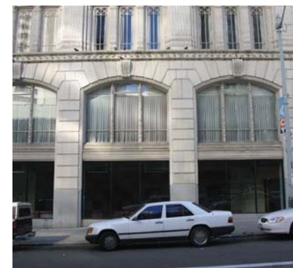
5. Looking east at the Eagles Temple Building (ACT Theatre).
