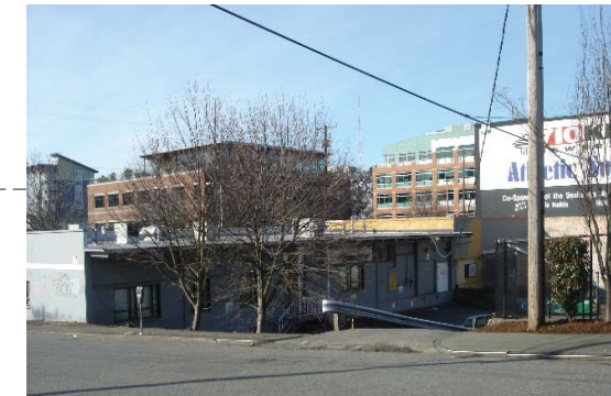
View of Site from SE
