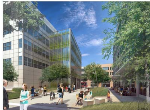
Figure 12: View from courtyard
