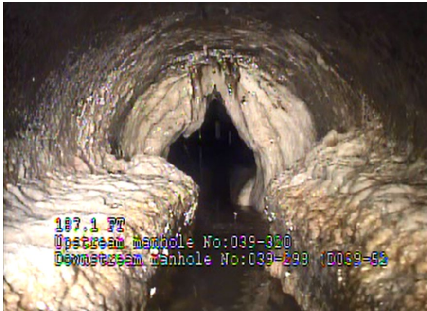
Figure 3-1. FOG Deposits in Sanitary Sewer Mainline – Pike Place Market Area
