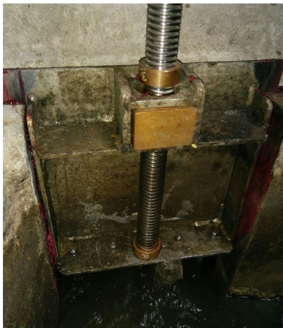
Figure 4-1. New Basin 99 Sluice Gate (left) and Actuator Motor (right)
