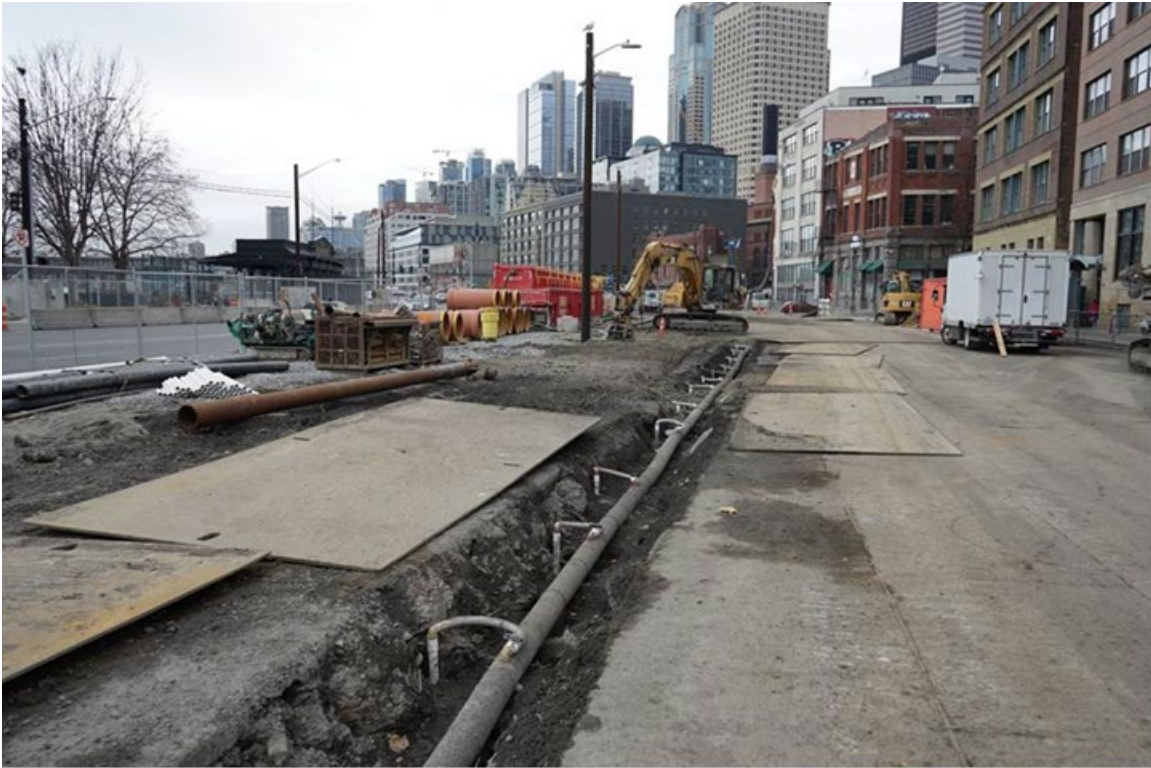
Figure 4-7. Central Waterfront Construction – Dewatering System
