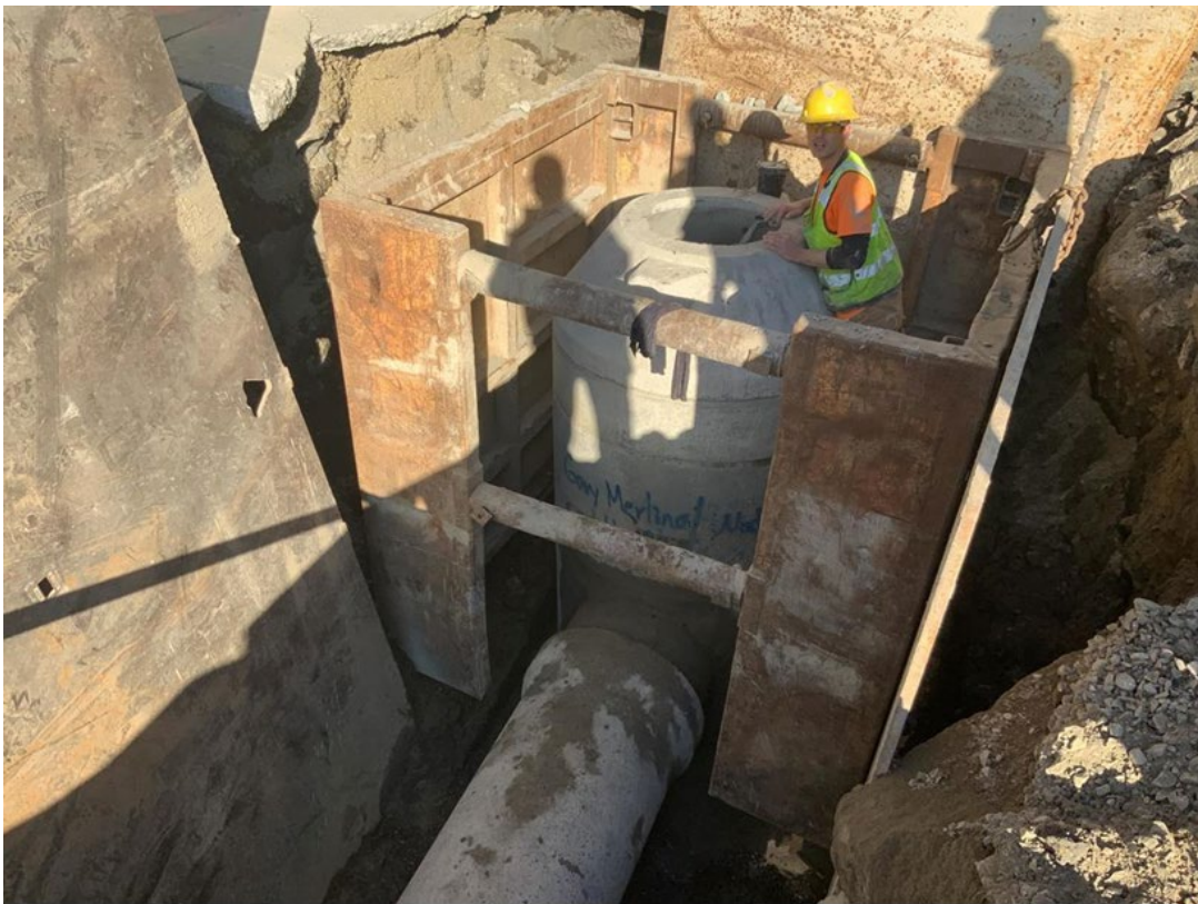
Figure 4-8. Central Waterfront Construction – Maintenance Hole Installation
