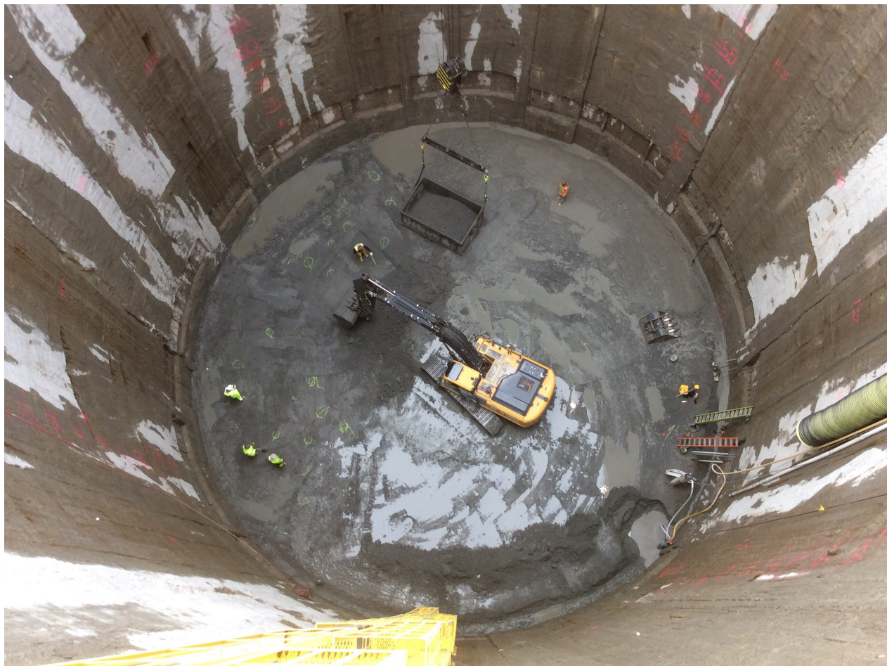
Figure 4-5. Drop Shaft Construction in Ballard
