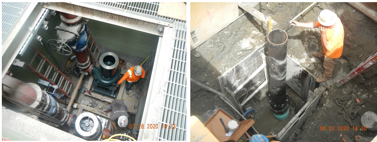
Figure 4-2. New Basin 60 pumps being installed (left) and New Basin 60 connection to King County trunk sewer (right)
