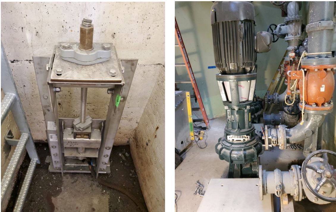
Figure 4-3. Installation of Basin 138 slide gate (left) and new higher capacity pumps (right)
