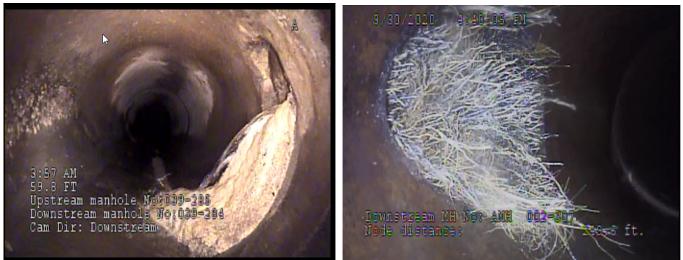
Figure 3-4. Private side sewer connections demonstrating visible FOG accumulations and impacts from root intrusion
