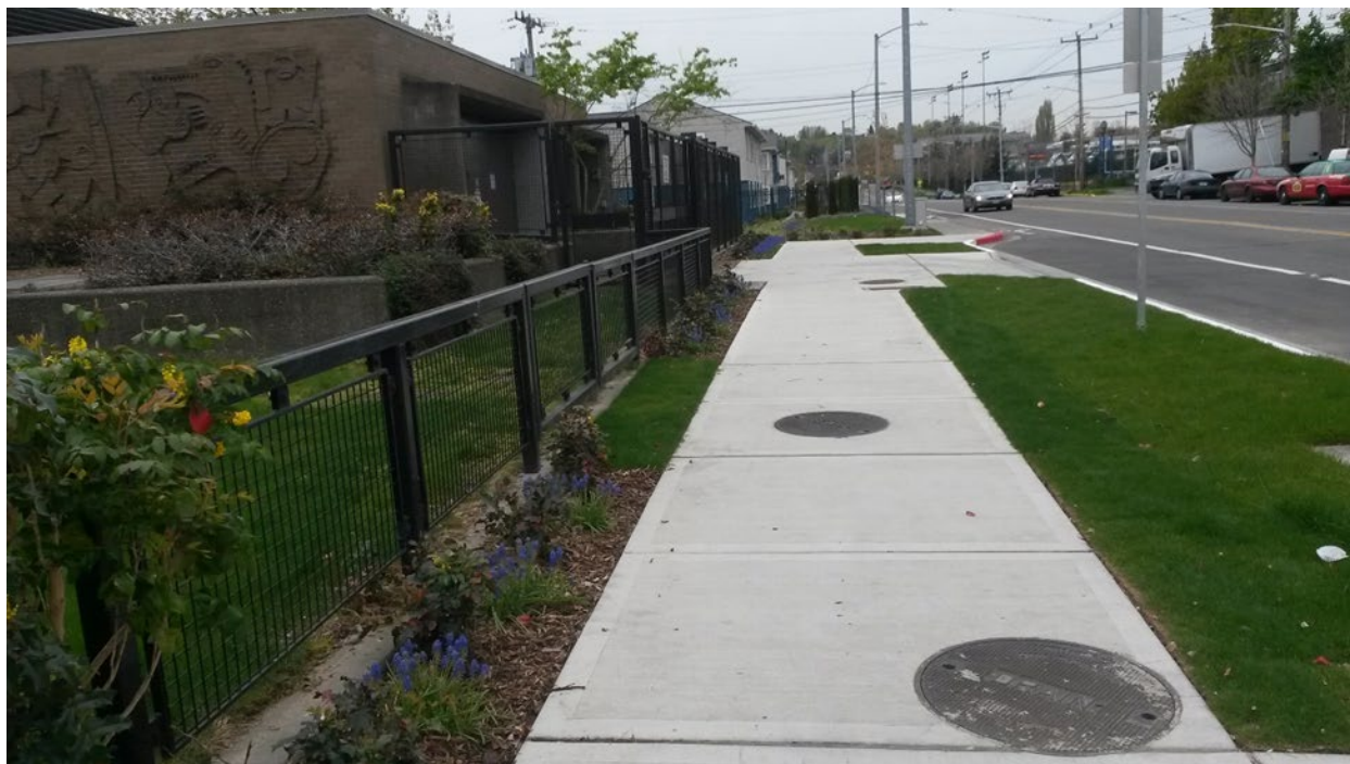
Figure 4-12. Completed 52 nd Ave S Combined Sewage Conveyance Project
