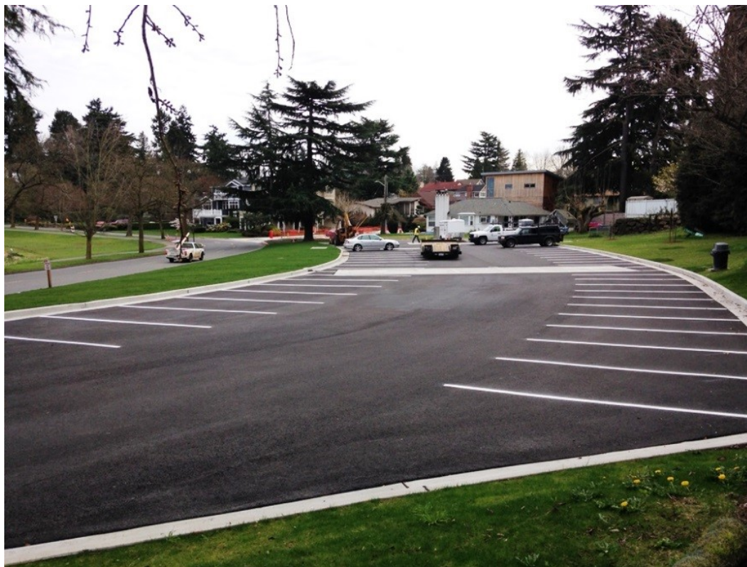
Figure 4-10. Completed Genesee CSO Storage Facility 9A
