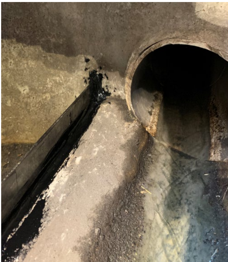
Figure 4-4. New Basin 140 smaller metal weir plate installed
