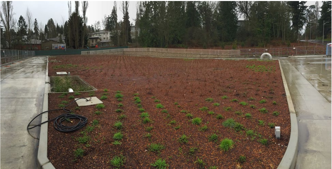
Figure 4-9. Completed Windermere CSO Storage Facility
