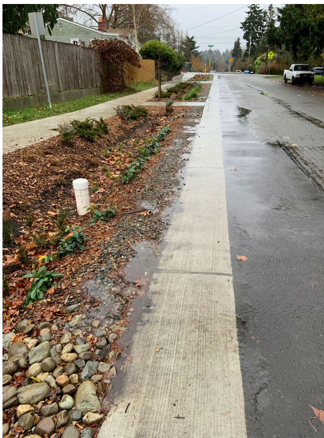
Figure 4-14. Completed 12th Ave NE Sidewalk and NDS Project
