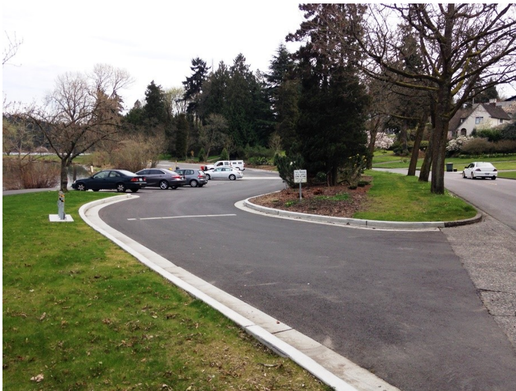
Figure 4-11. Completed Genesee CSO Storage Facility 11A
