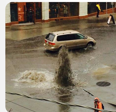
Extreme rainstorms in Seattle increased by 30% between 2003 and 2018. Extreme rain events are increasing the need for climate-resilient drainage and wastewater infrastructure.
