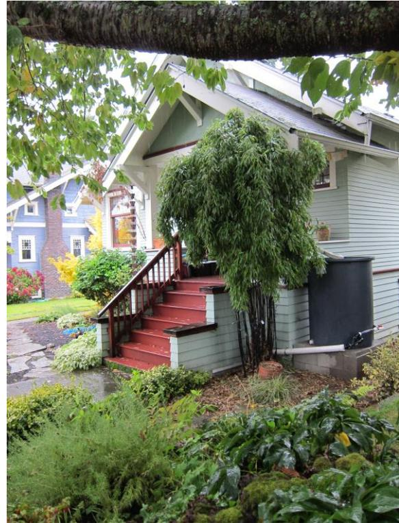
**Figure 4-9. Raingarden (left) and Cistern (right)**
