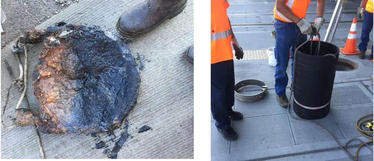
Figure 4-1. Removed Flap Gate (left) and New Backwater Valve (right) in Basin 107
