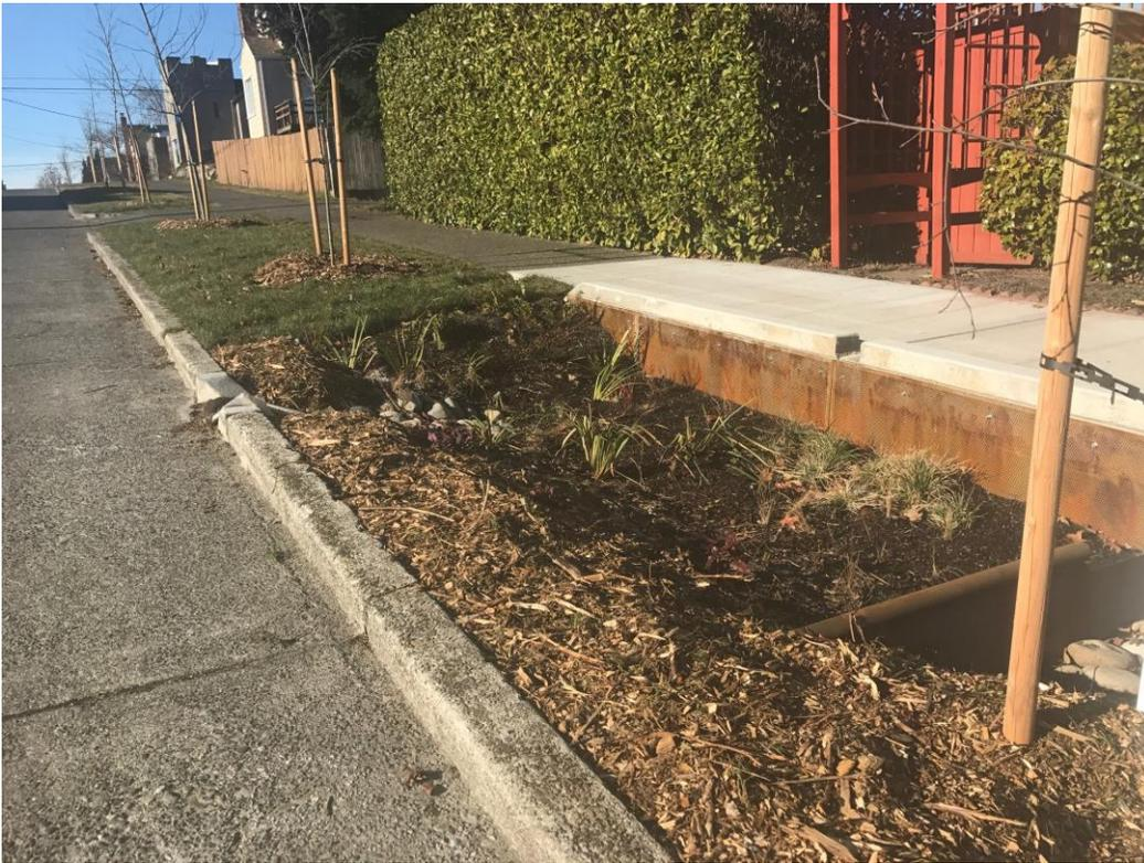
**Figure 4-3. Ballard NDS 2015 Modular Soil Cells**
