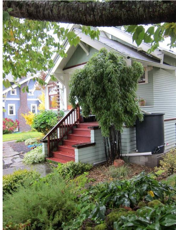
**Figure 4-2. Raingarden (left) and Cistern (right)**
