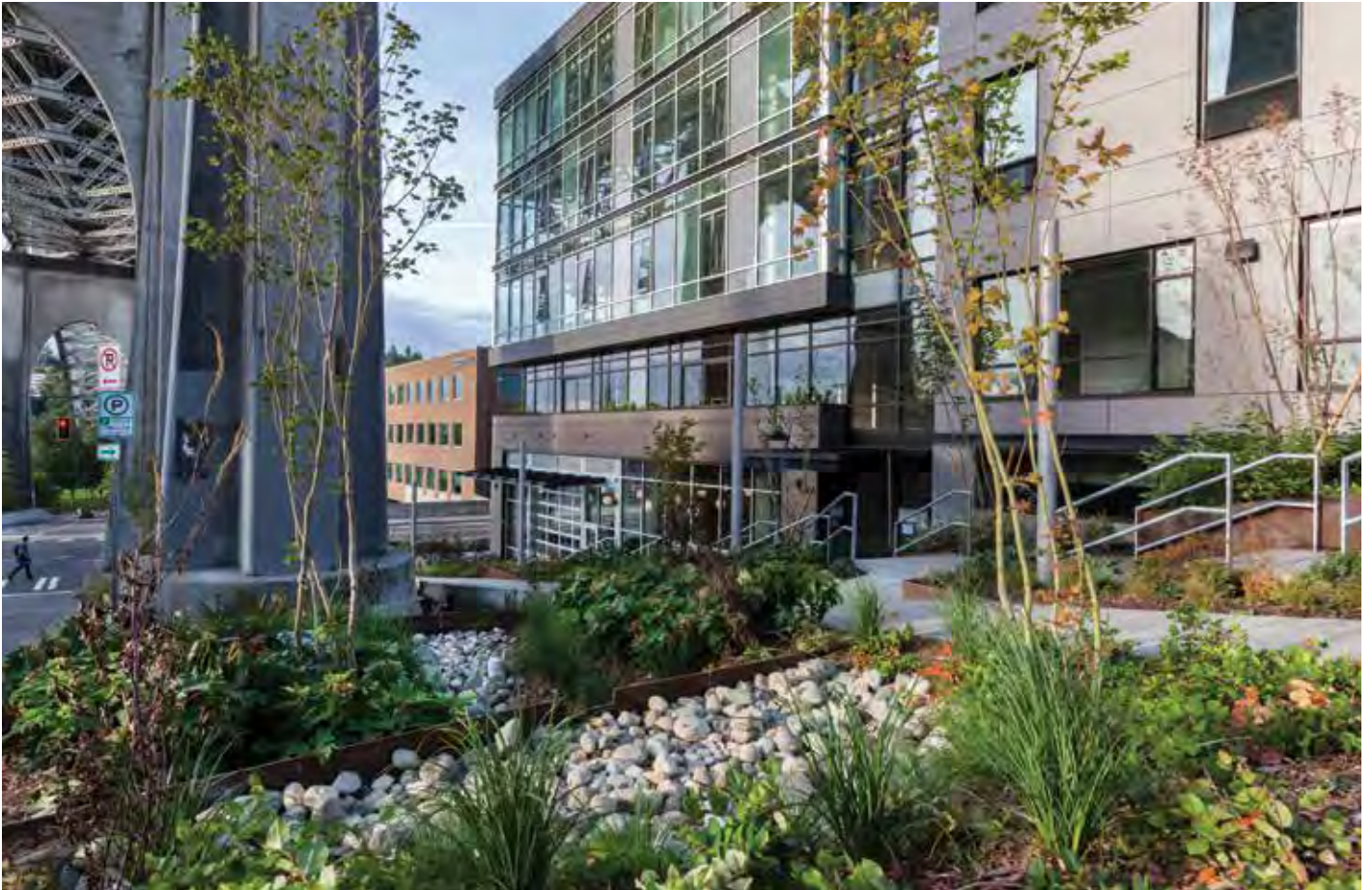
Imagine a city where we are capturing and treating road runoff from all our bridges!
