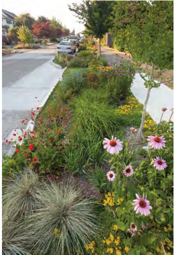
Barton Basin parking strip transformed into a roadside rain garden.
