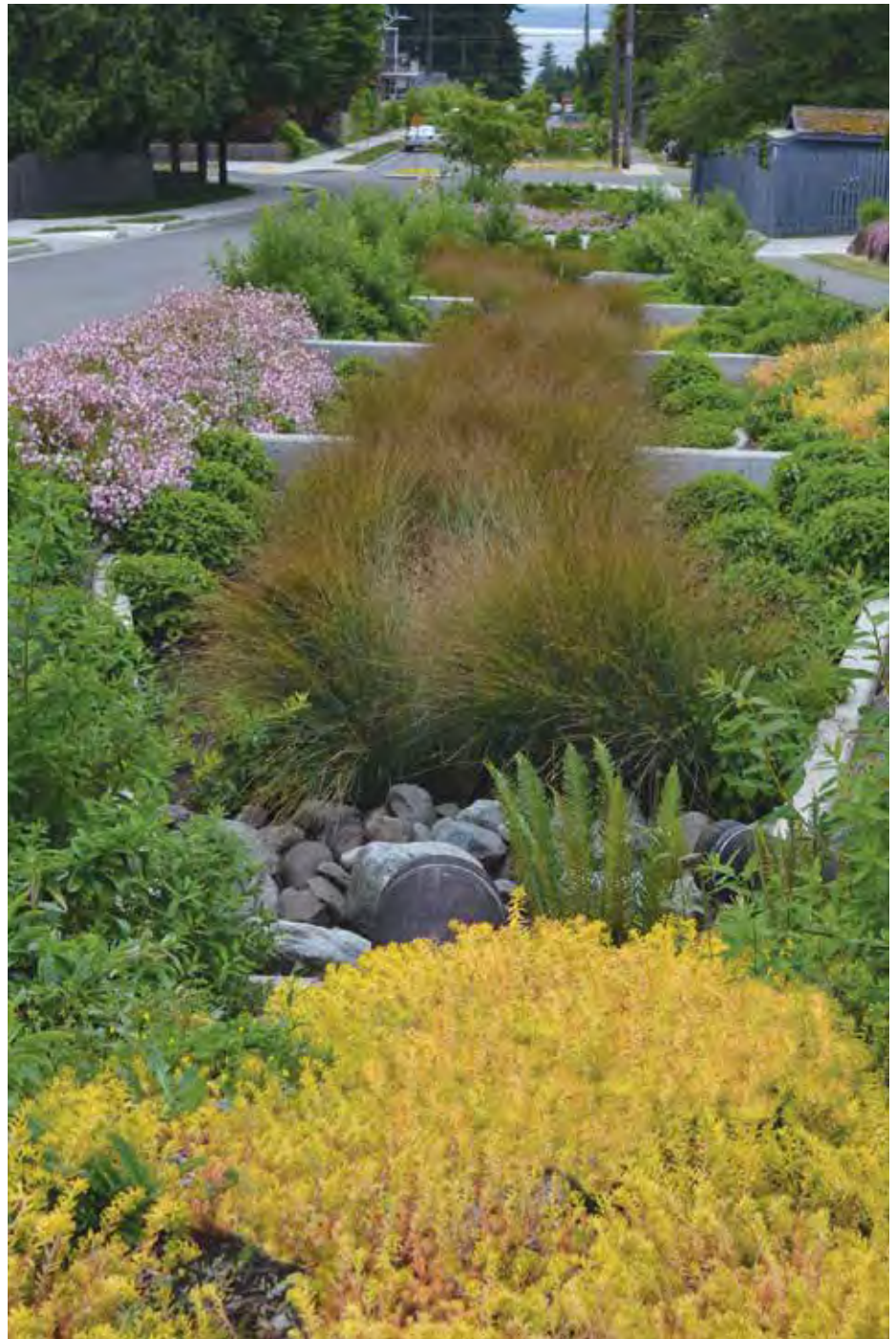
Venema Creek neighborhood bioretention swale.
