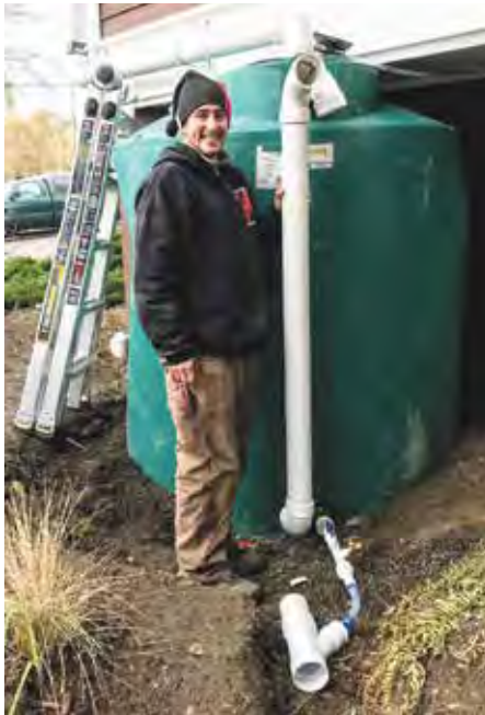
A stormwater cistern being installed by DIRT Corps.
