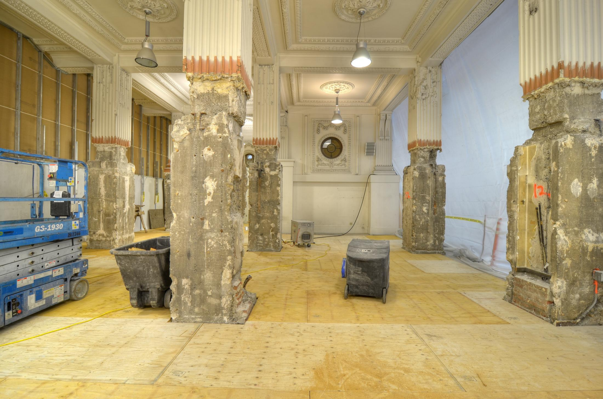
Original structural supporting column without their gypboard panels in the pre-ticketing area.
