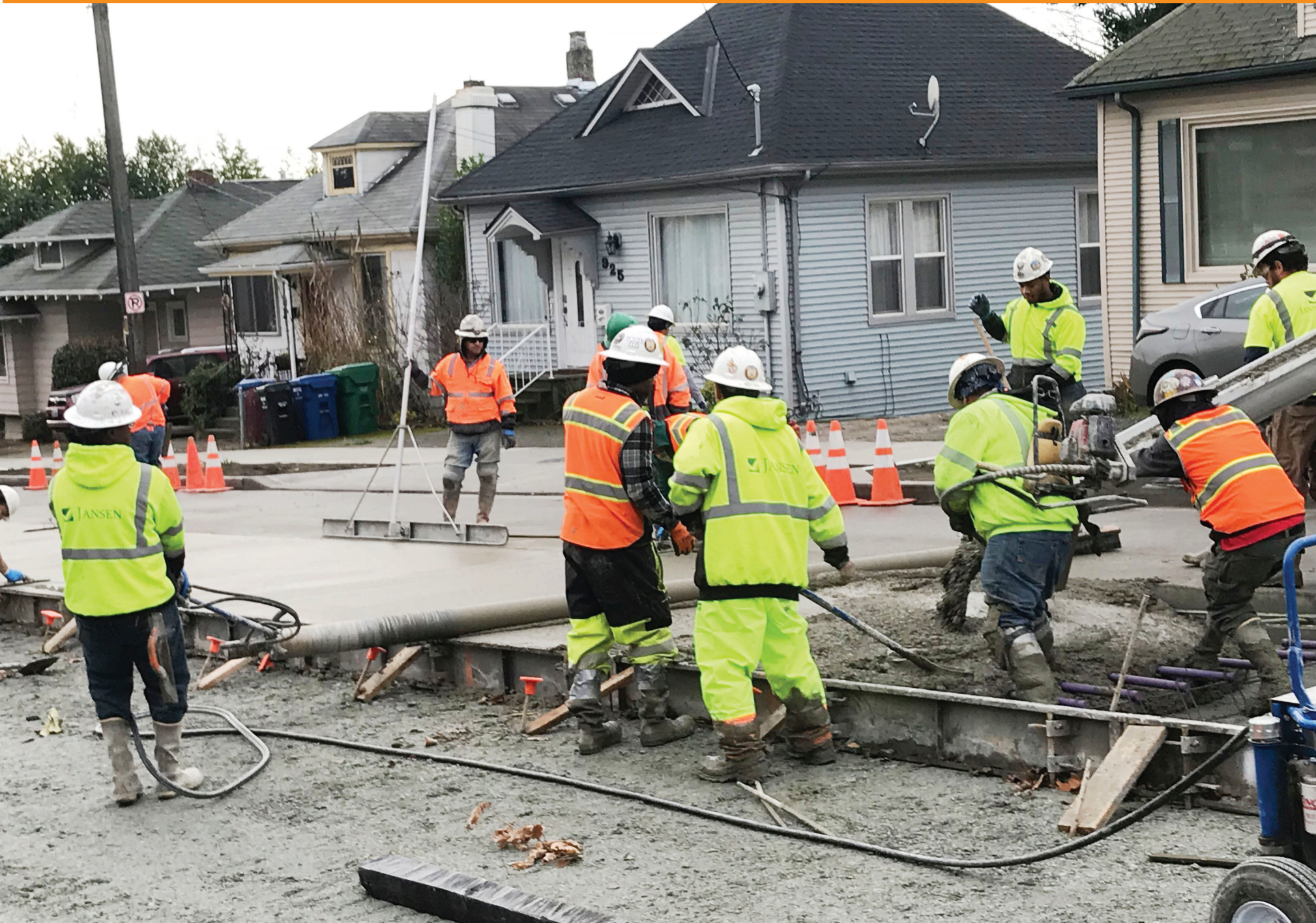
Full depth concrete work
