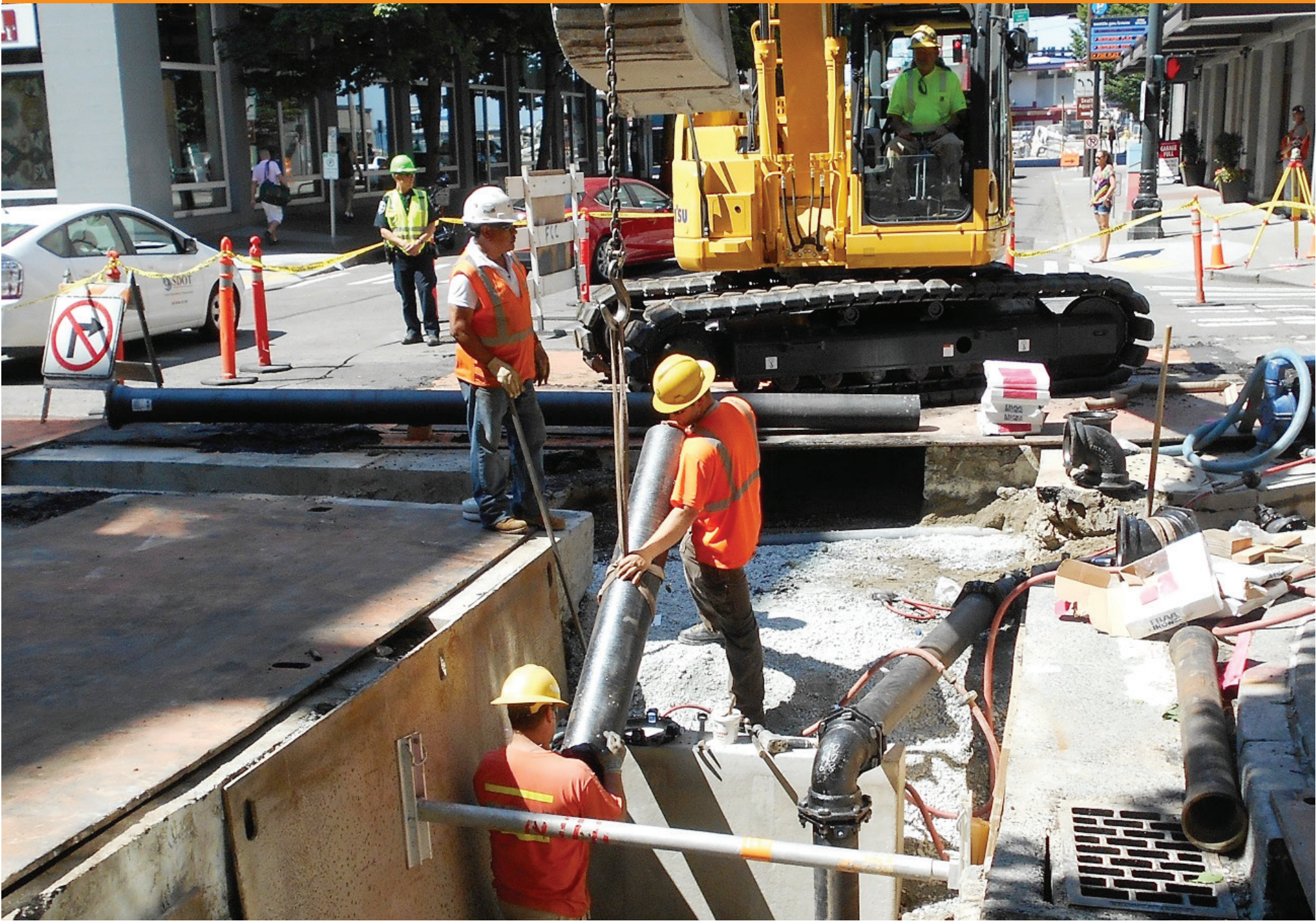
Replacing the water main
