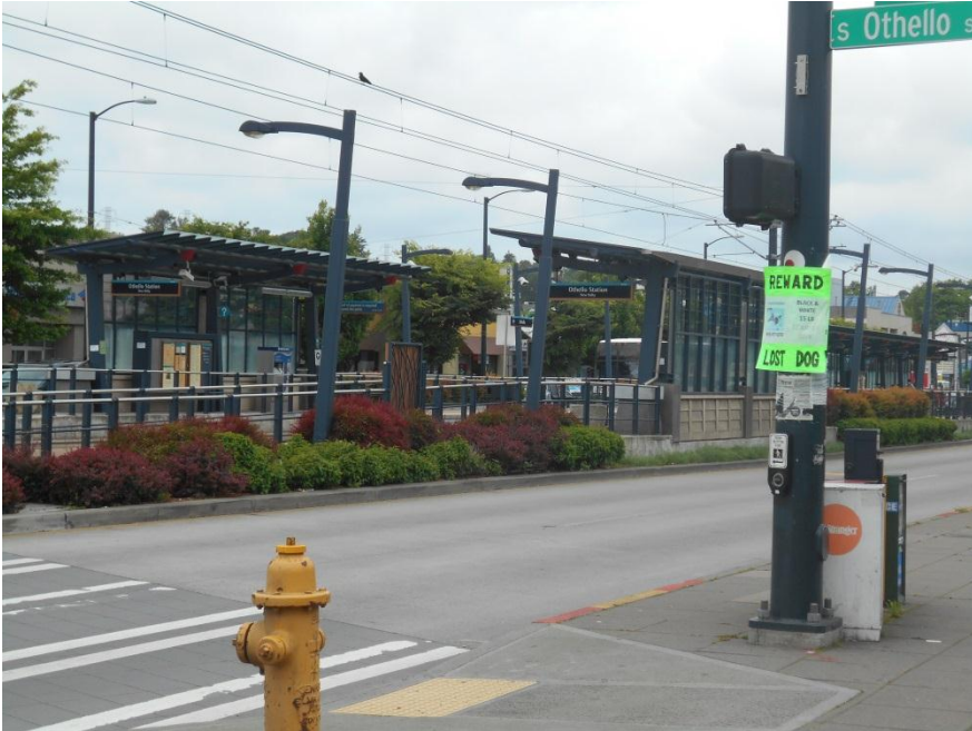
Othello Light Rail Station
