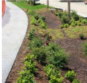
**Figure 16: Stormwater Surface Treatment**
