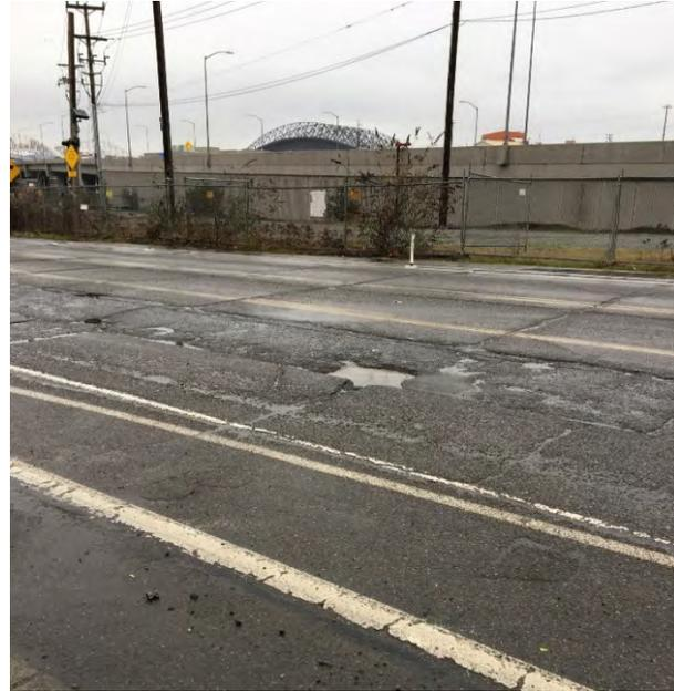
**Figure 8: Deteriorated Roadway Conditions on East Marginal Way S**
