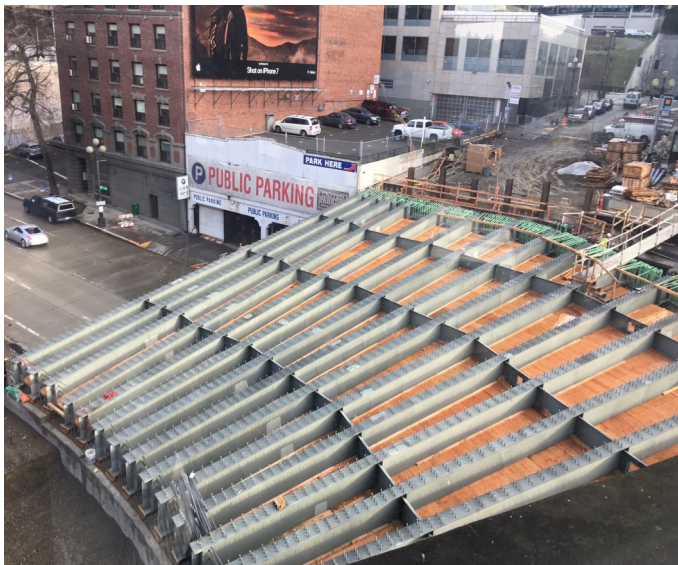
View after setting of new girders.
