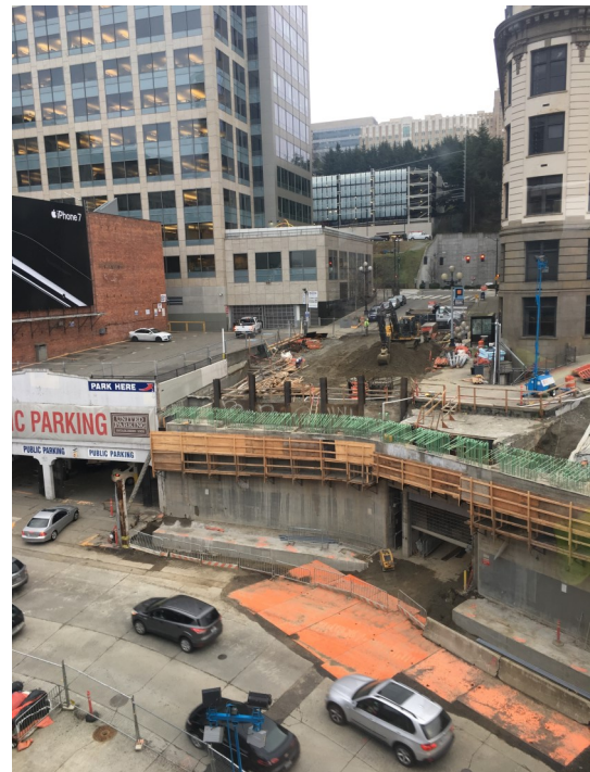
View before setting of new girders.
