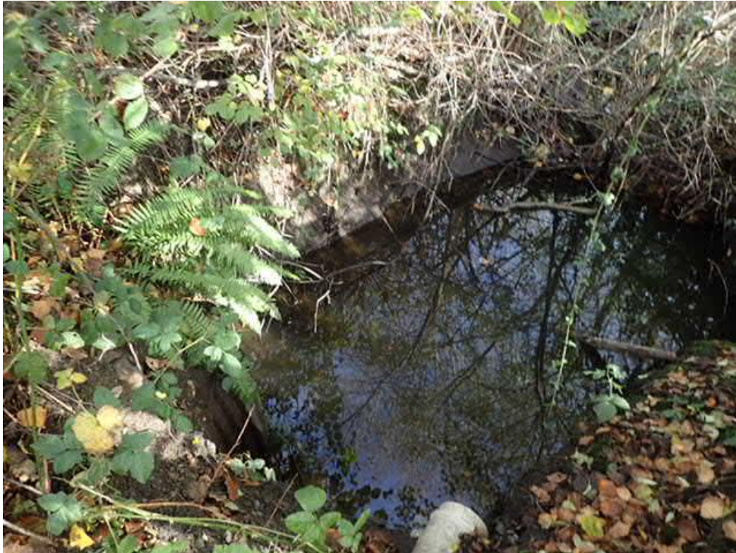
Photo 1: Culvert Outfall to Western End of Watercourse 5 – Looking Northeast
