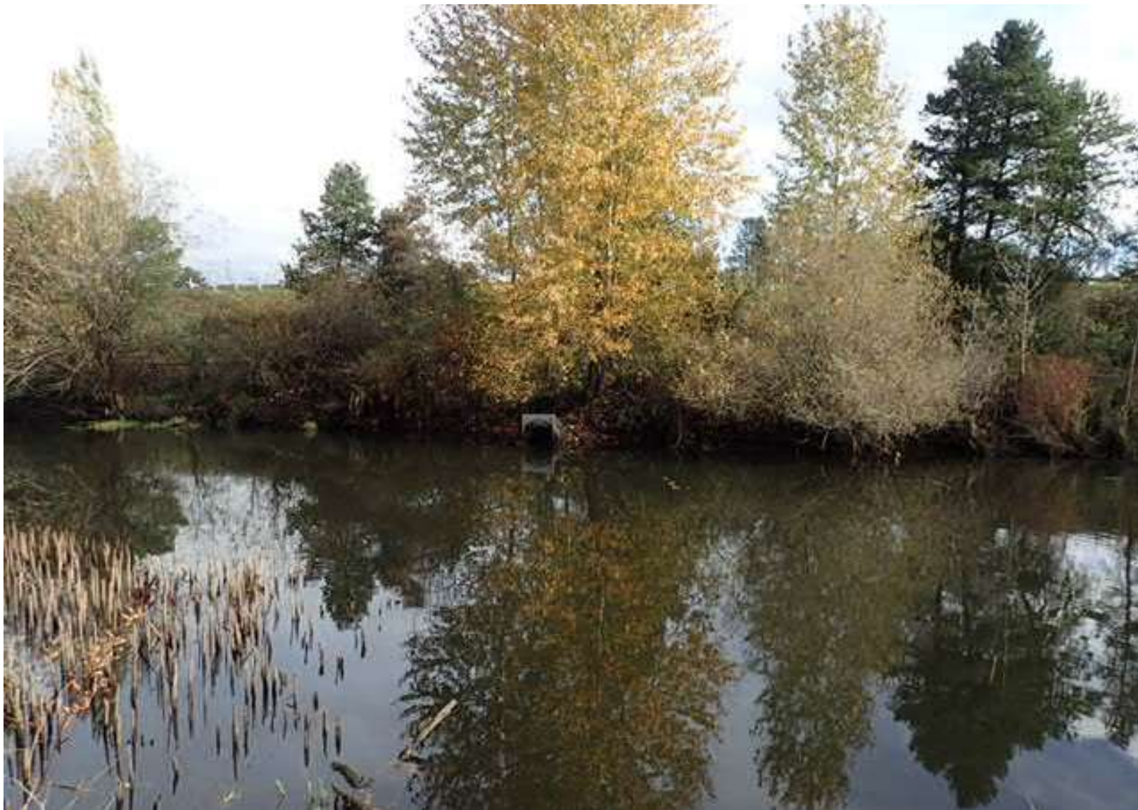
Photo 5: Wetland 6 (Surge Pond) Outlet Culvert under I-5 – Looking East-Northeast
