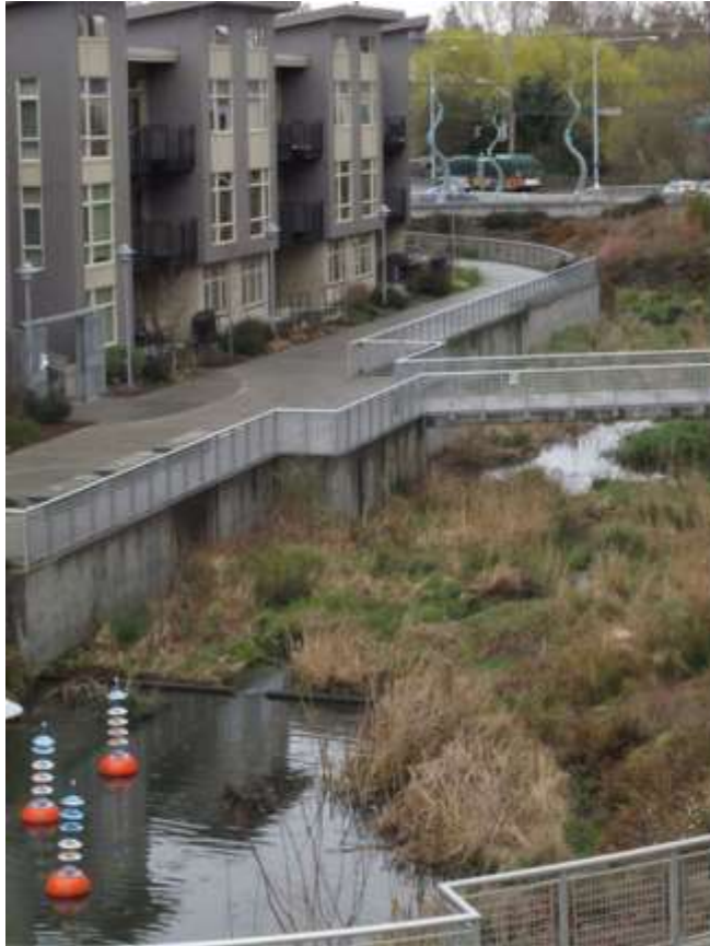
Photo 7: Water Quality Facility at Thornton Place
