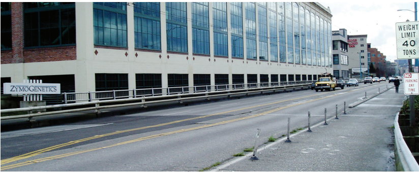
Fairview Ave N bridge directly next to the historic Lake Union Steam Plant Building.
