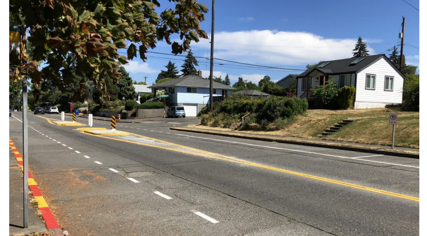
16 th Ave SW and SW Elmgrove St median islands
