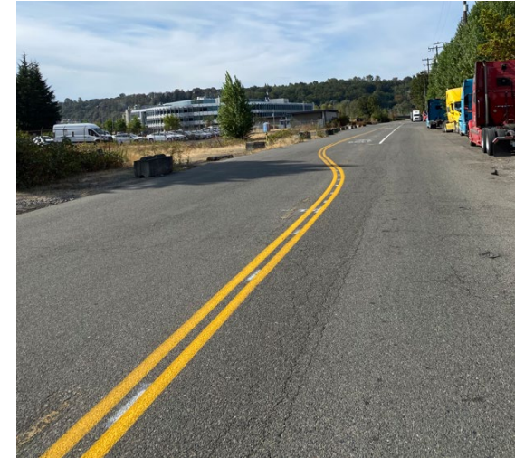
Diagonal Ave S restriping
