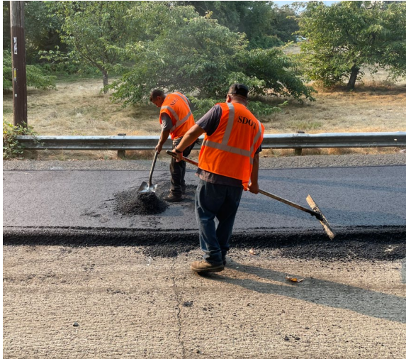
Repaving California Ave SW
