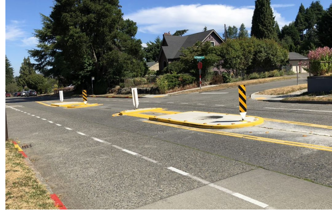
16 th Ave SW and SW Elmgrove St median islands
