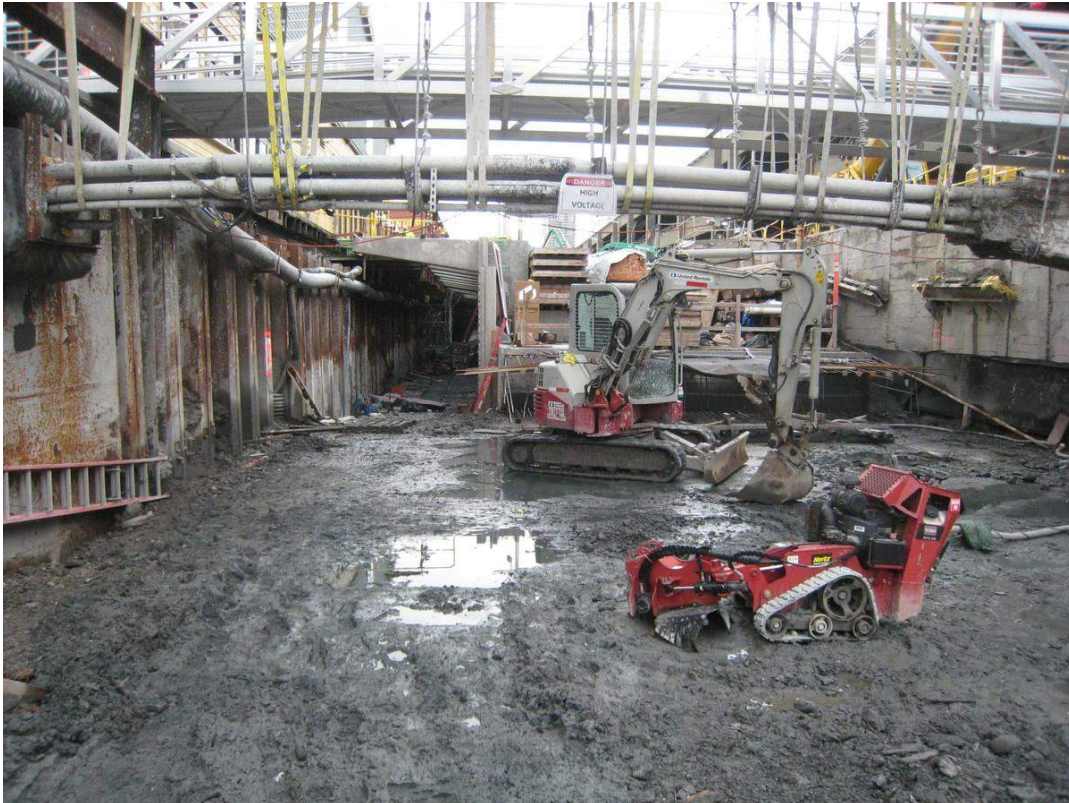
Figure 2. Electrical duct bank spanning jet grout work zone, pedestrian bridge beyond
