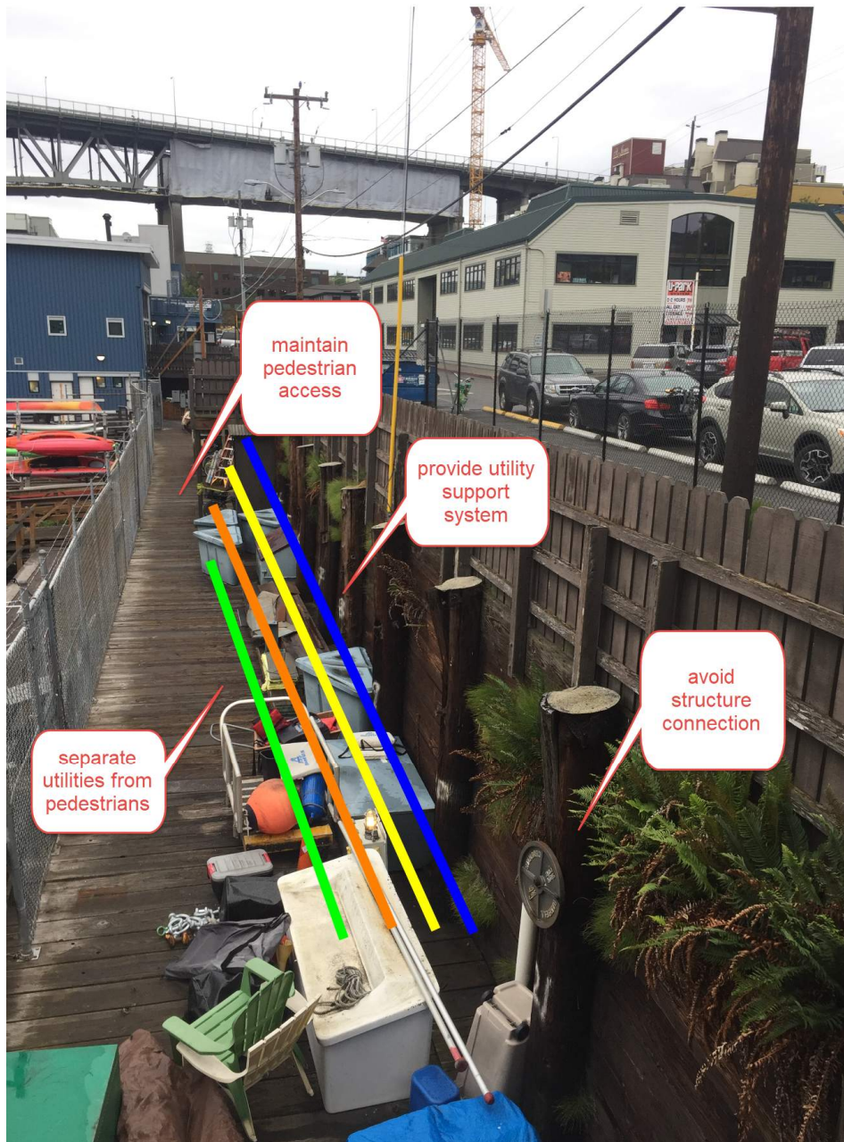
Figure 3. Temporary utility requirements across the marina zone
