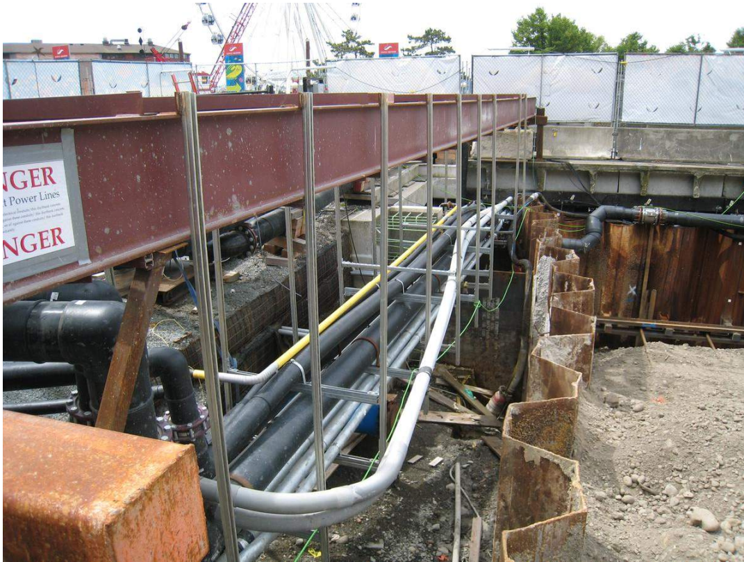
Figure 1. Example temporary utility support
