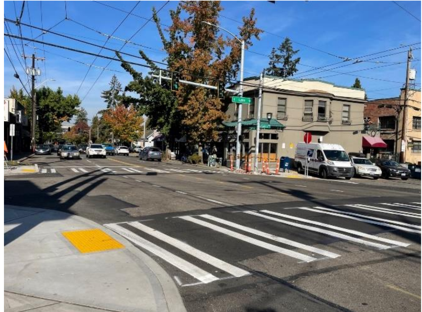
New signal at E Lynn St and 23 rd Ave E
