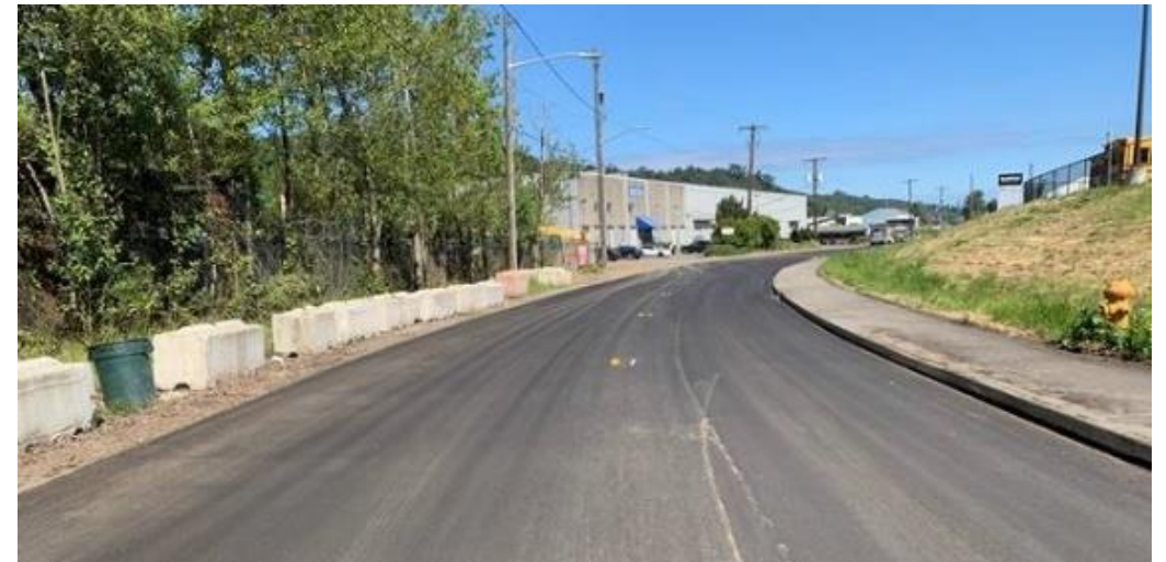
Before (top) and after (bottom) paving on Occidental Ave S between S Kenyon St & S Sullivan St.
