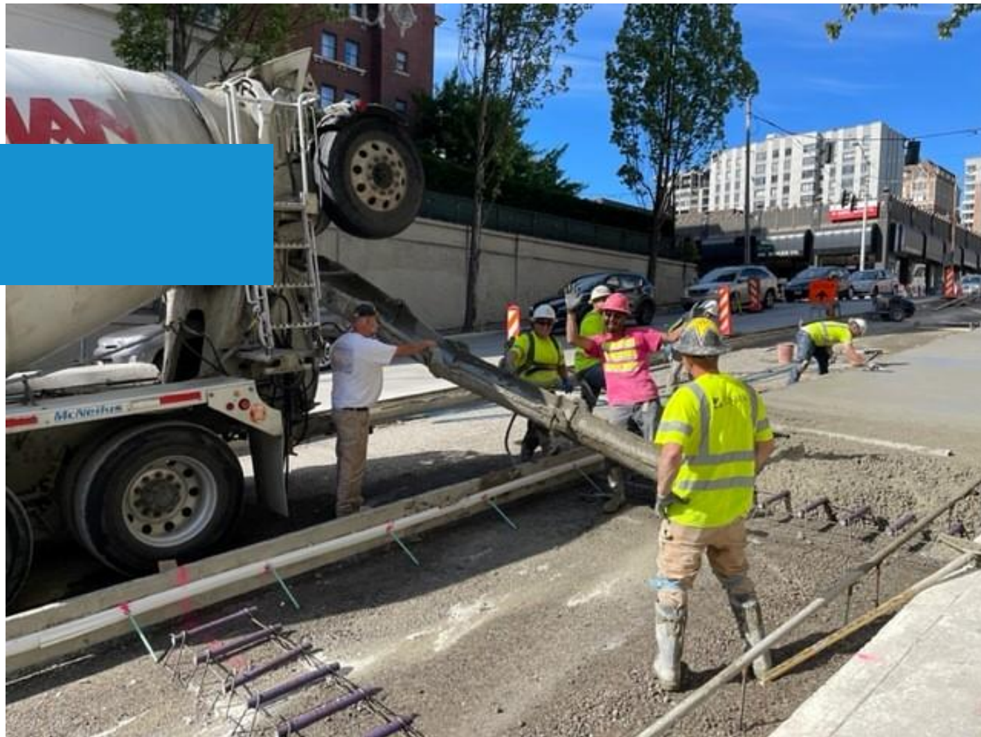
Paving on Madison RapidRide G Line project.
