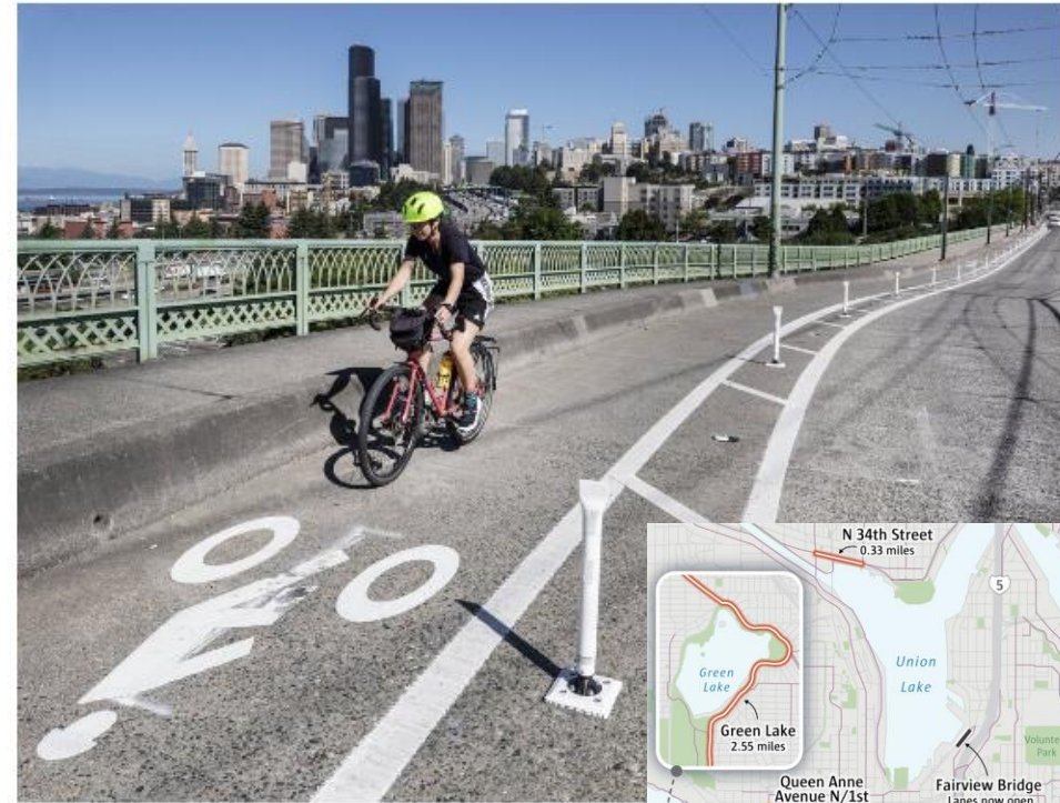
A rider climbs the slight hill on Dr. Jose P. Rizal Bridge. New bike lanes on both sides of the bridge connect
