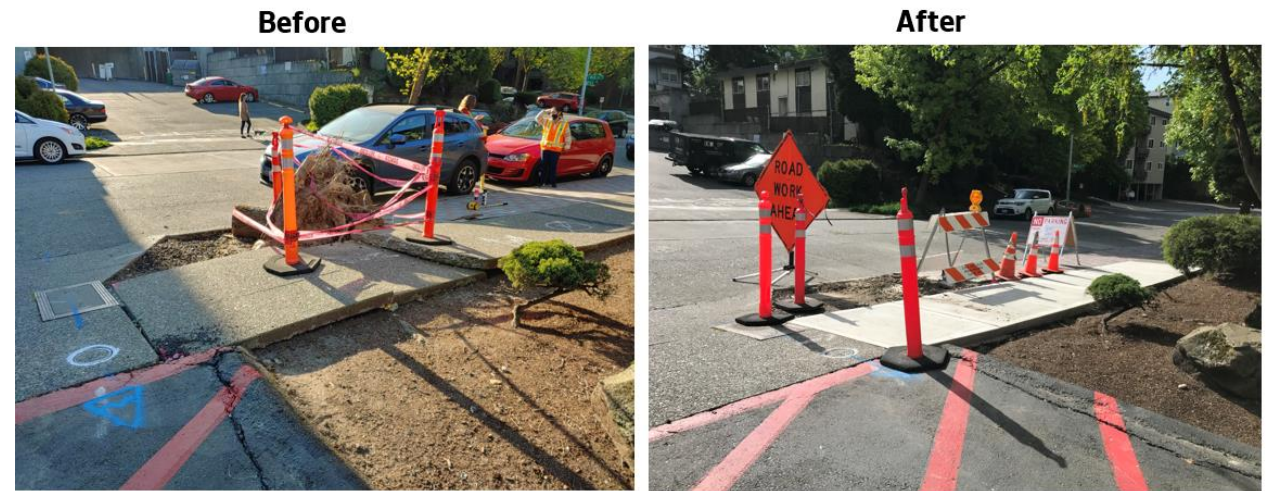
Sidewalk repair funded by the Levy in Q2 on 22 nd Ave S.
