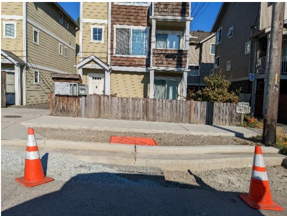
New sidewalks under construction on Greenwood Ave N.
