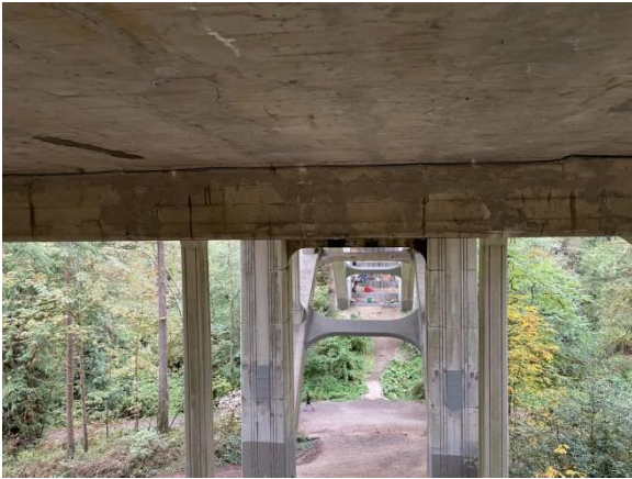
One bridge spot repair we completed this quarter was filling cracks on the Cowen Park Bridge with epoxy.
