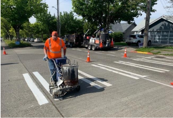
Restriping the crosswalk at 16th Ave SW and SW Findlay St.
