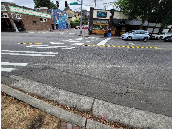
New hardened centerline on Rainier Ave S.
