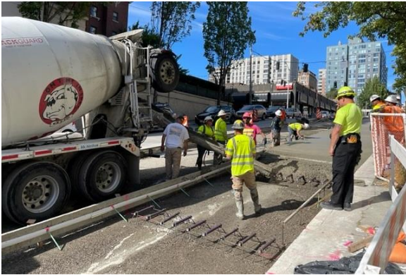
Repaving underway as part of the Madison RapidRide G Line project.
