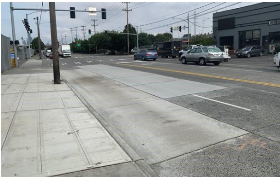
Before (top) and after (bottom) paving on 4th Ave S between Industrial and S Spokane streets.
