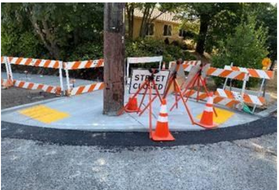
New curb ramp under construction on Latona Ave NE and NE 52nd St.
