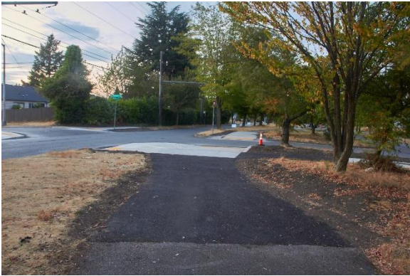
Beacon Ave S repaving.
