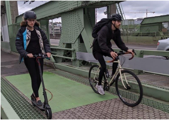
The University Bridge.
