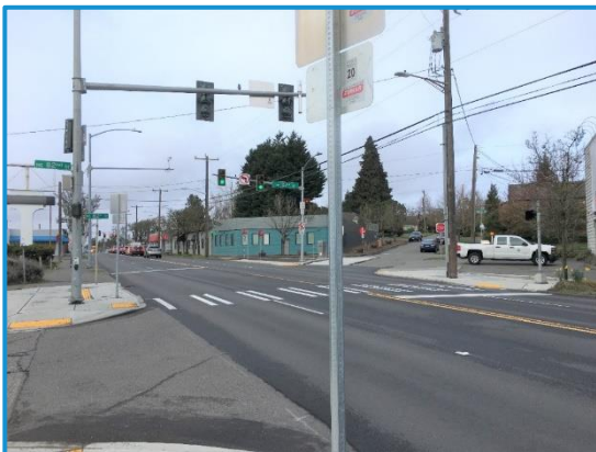
New curb ramps and crossing at the intersection of Lake City Way and NE 82nd St.
