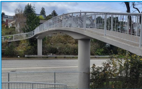
SW Andover St Pedestrian and Bicycle Bridge.
