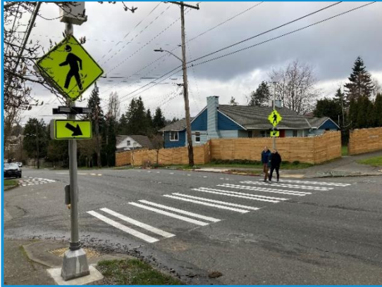
The NE 65th St and 28th Ave NE intersection, improved as part of the NE 65th St Pedestrian Safety Enhancements Project.
