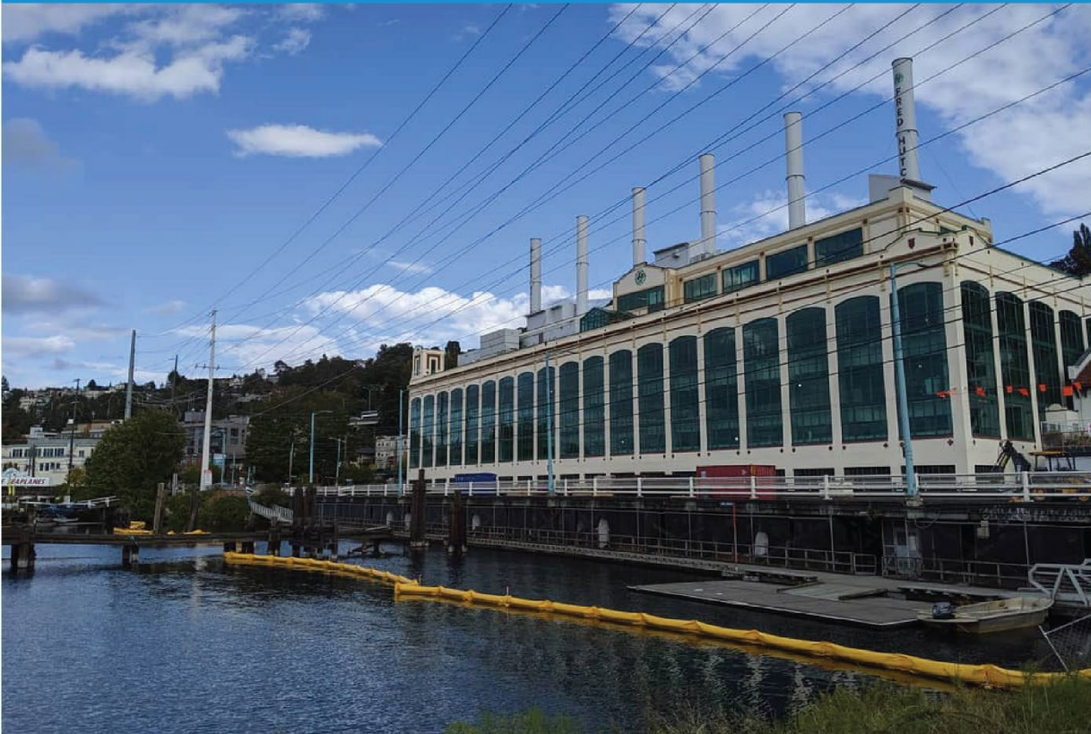
The Fairview Ave N Bridge.
