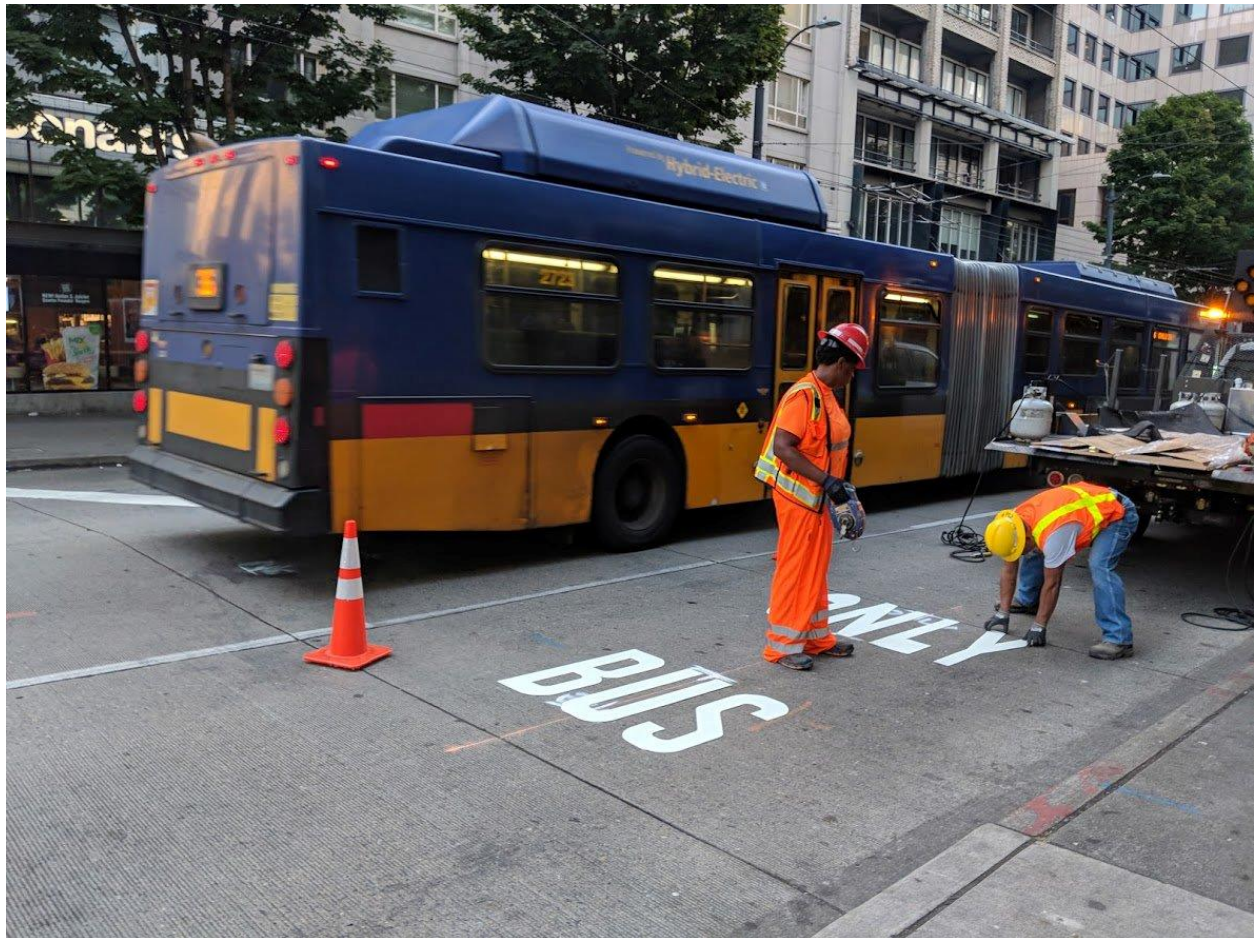
Crews working to install red bus lanes to keep transit moving through critical areas around town
