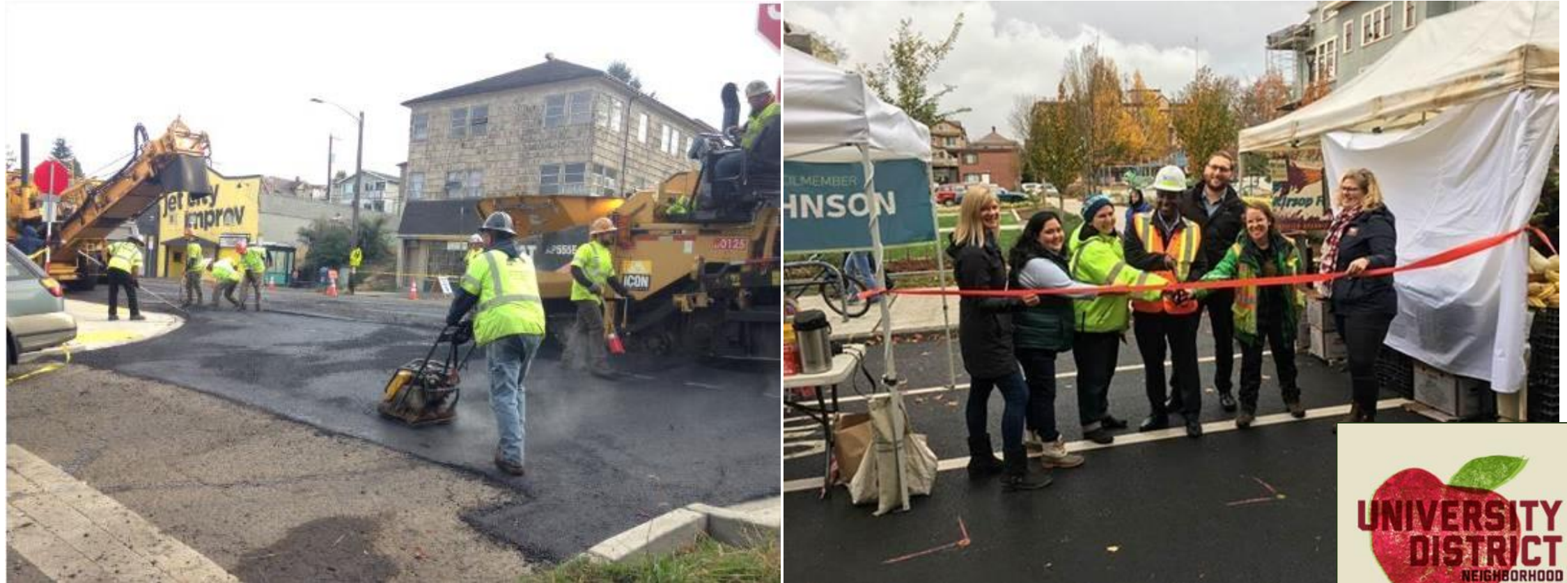
Paving construction and project ribbon-cutting event for University/Cowen paving project.
