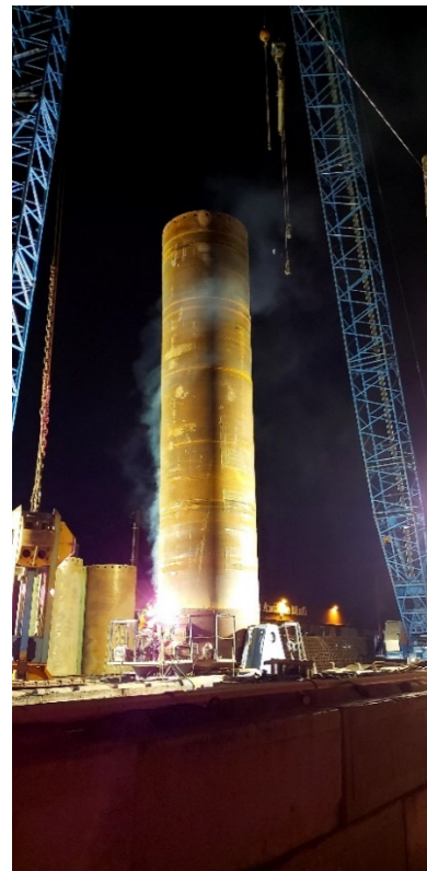
Crews weld shaft casing for Lander Bridge
