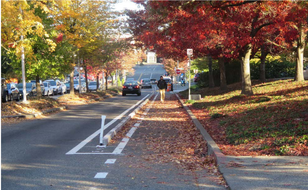
Low-cost sidewalk on 3rd Ave NE
