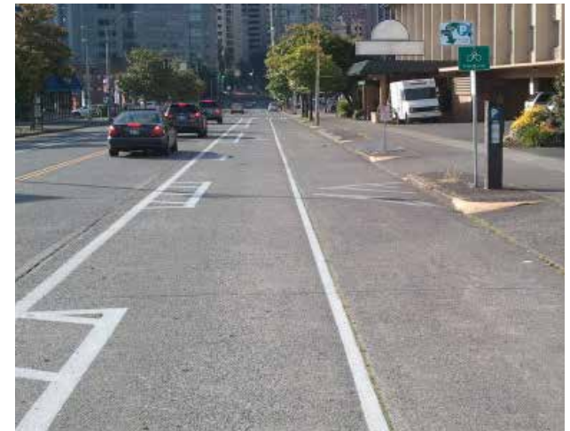
Existing 7 th Avenue Bike Lane, looking south
