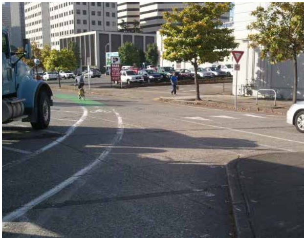
Difficult Bike / Vehicle Intersection, south of Denny
