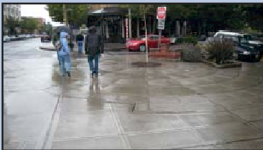
Neighborhood Street Fund project along Ballard Ave
