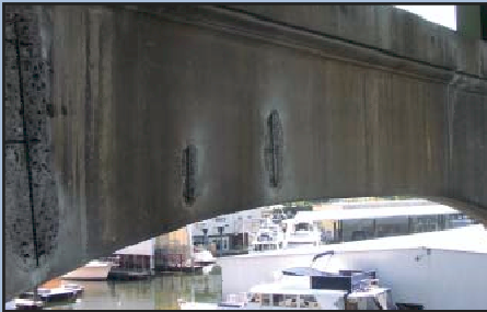
Bridge repair on Ballard Bridge
