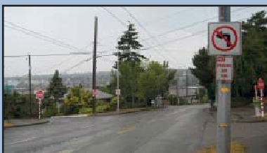
High collision location improved at NW Market St and NW 49th St
