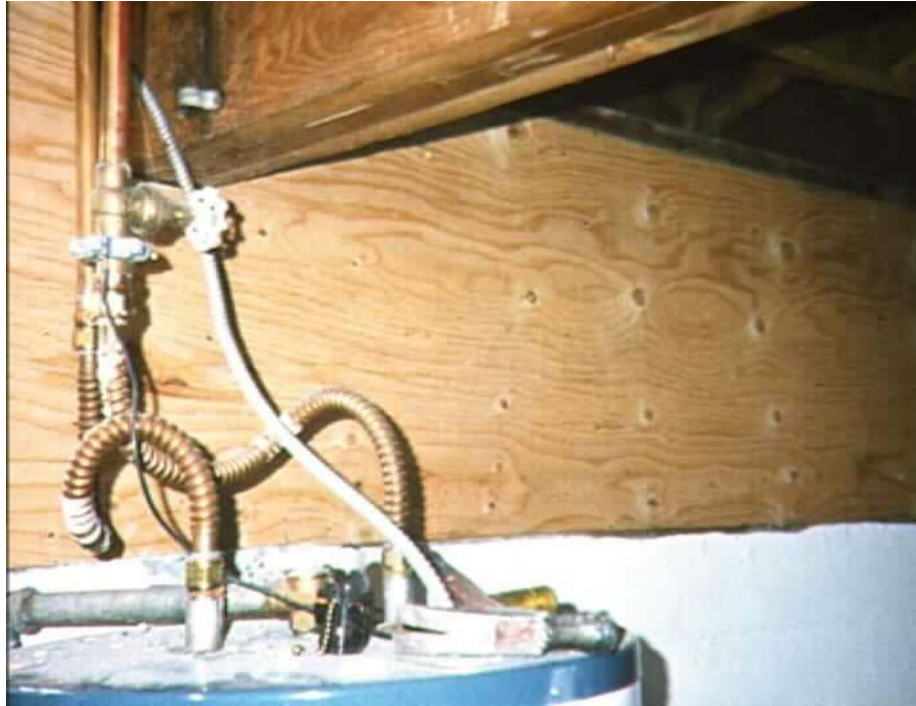
Figure 11 Refer to Drawing Detail 2d to determine how to cut-out a section of the structural panel to accommodate piping, etc. (Photo from Ben Emam)
