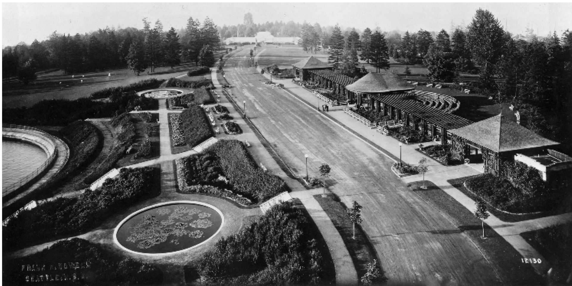
1913 PARK VIEW (BAND PAVILION WITH SEATING ON RIGHT; DEMOLISHED IN 1931) ORIGINAL BAND PAVILION
