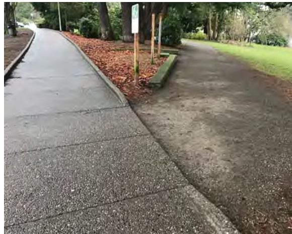
SIDEWALK TO GRAVEL TRANSITION
