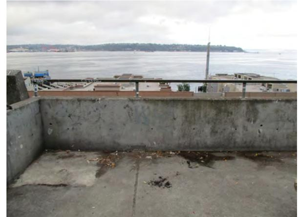
Concrete Stem Wall at Guardrail
