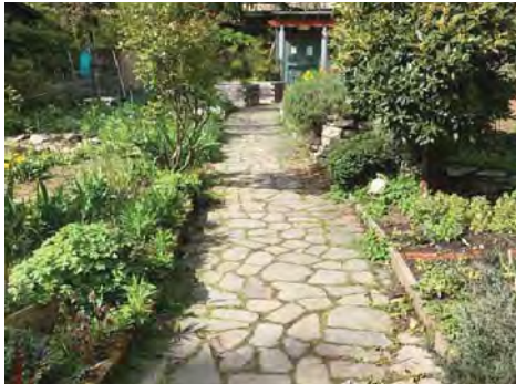
Reset pavers in mortar to provide greater accessibility
